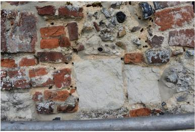
**Photograph 7** Detail of wall showing numerous masonry bee burrows. Photograph taken facing north-east.
