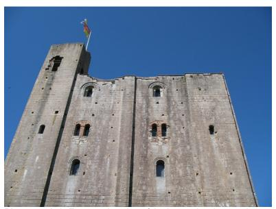
**Photograph 8** Eastern elevation of the keep, showing repairs undertaken to other windows, including some with apparent collapse below. Photograph taken facing south-west.
