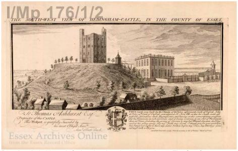
**Drawing 1** 1738 north-facing drawing showing the keep. The first-floor entrance and scar delineating the presumed top of the fore-building are both present, but no infilling or repair is visible. Image courtesy of Essex Record Office (ERO) I/Mp 176/1/2.
