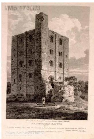
**Drawing 3** 1810 south-east facing drawing of the keep. No infilling or repair visible, and the window opening above the first-floor entrance clearly has a carved surround. Image courtesy of ERO I/Mp 176/1/3.
