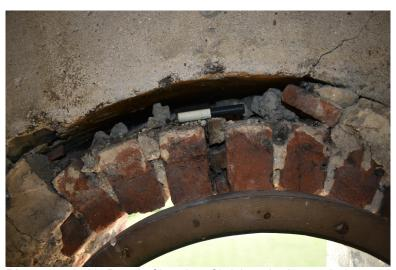
**Photograph 10** Detail of interior of brick arch above window, showing gap between it and the mortar and flint above. Photograph taken facing south-west.
