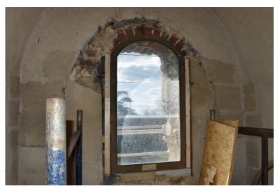
**Photograph 9** Interior of window in section of wall, showing exposed brick arch. Photograph taken facing west.
