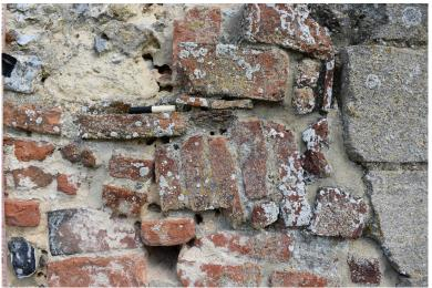
**Photograph 6** Detail of reused Tudor brickwork in make-up of wall, bonded in cement. Photograph taken facing north-east.
