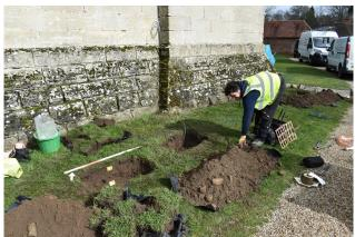
**Photograph 2** Excavation of pads for lightning conductor in progress. Photograph taken facing north.
