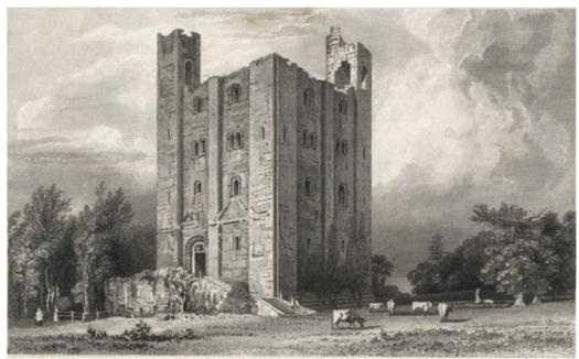
**Drawing 6** 1831 north-east facing drawing, showing the infilling/repair clearly for the first time. Also note the window above the first-floor entrance is now shown as smaller than in previous drawings, without a carved surround. Drawing courtesy of ERO I/Mp 176/1/24.
