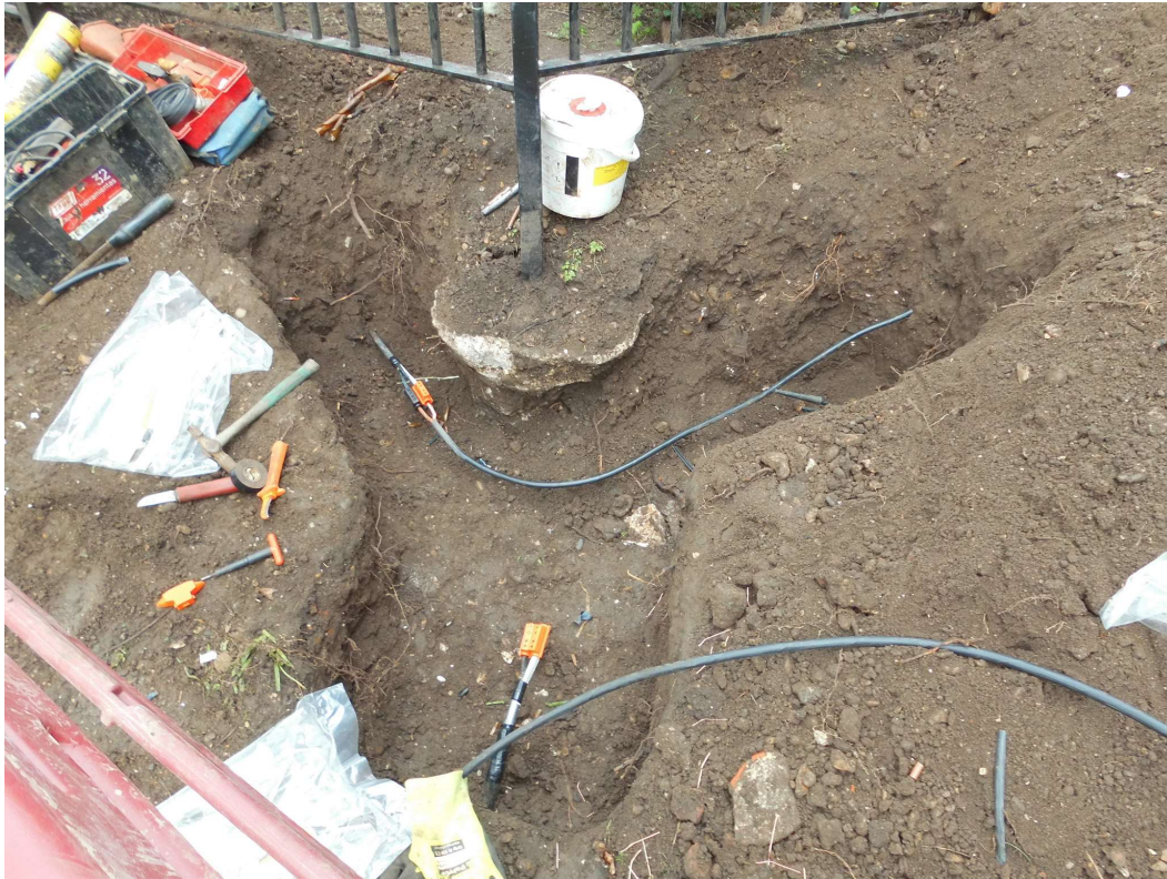
Photograph 1 The full extent of groundworks, looking southeast
