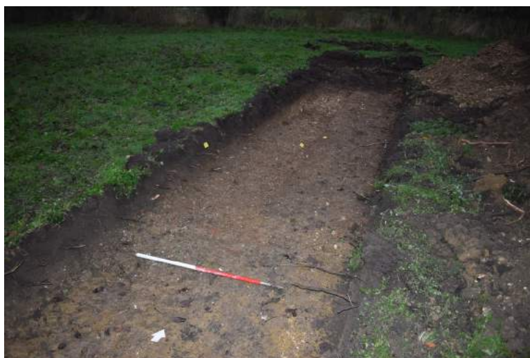
Photograph 3 Northern end of T2, showing section excavated through L5 and the metallised surface L7 beneath. Photograph taken facing north-west.
