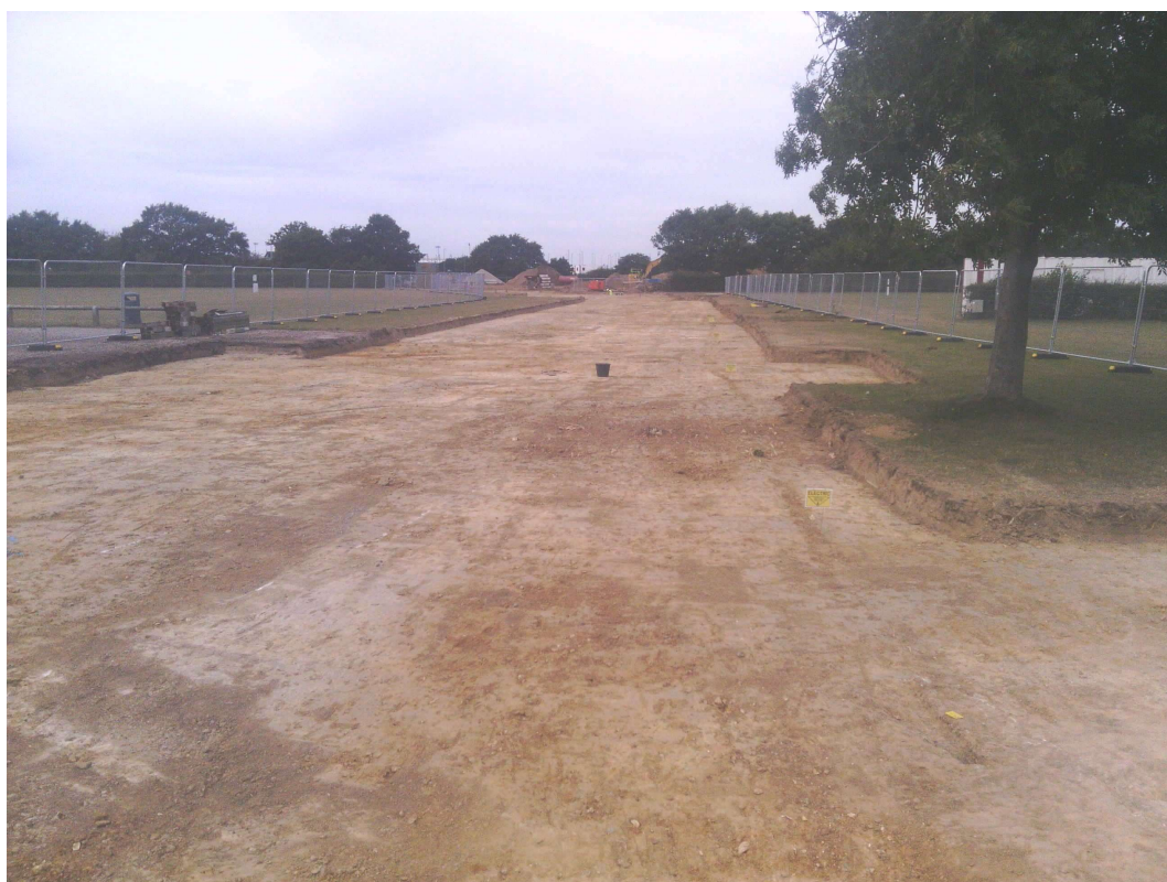
Photograph 2 Road strip, looking north-west
