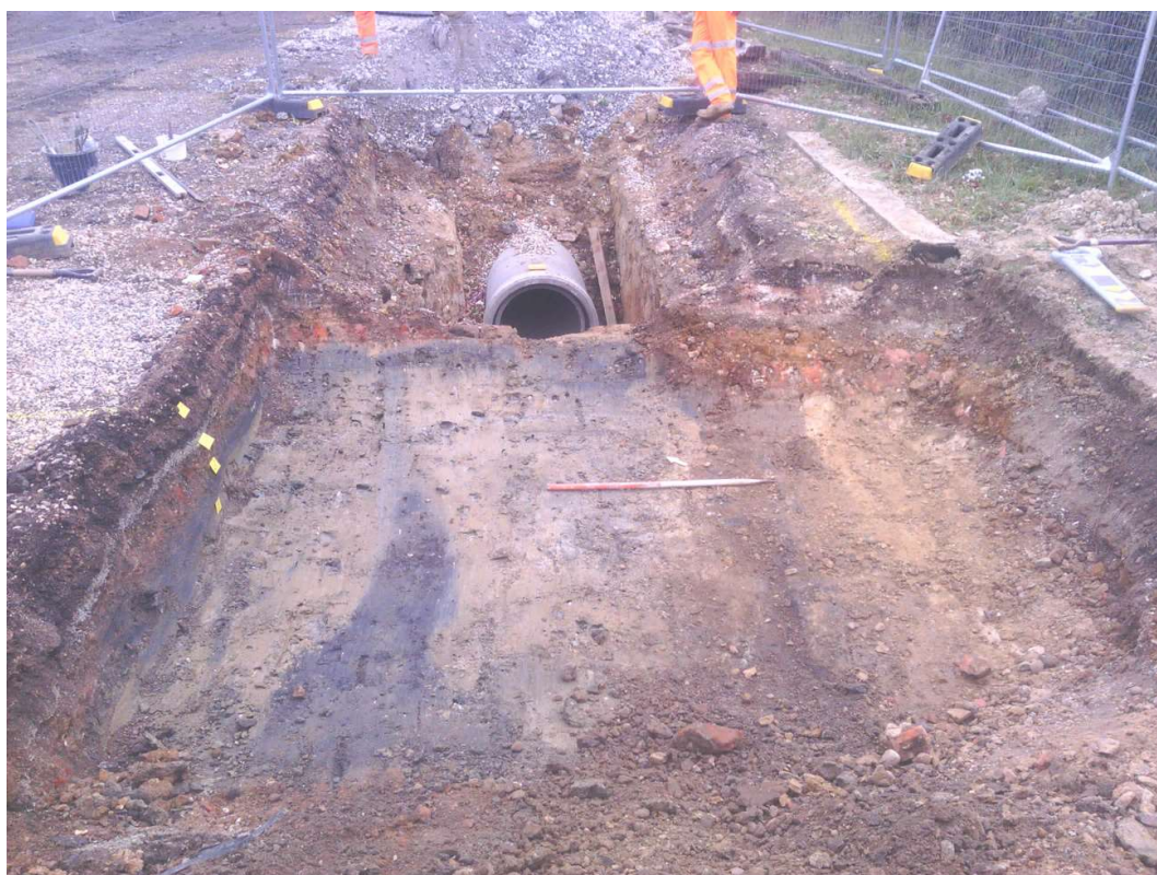
Photograph 8 Drainage trench strip through the car park, looking north-east
