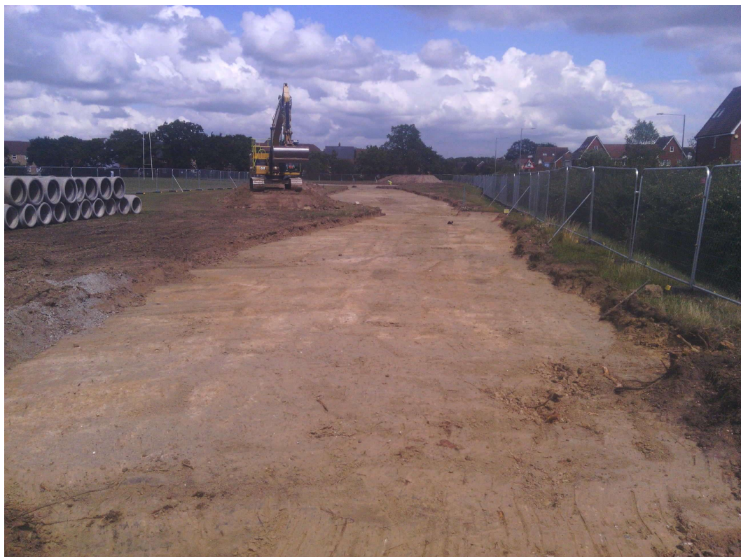
Photograph 7 Swale and drainage trench strip, looking north-east
