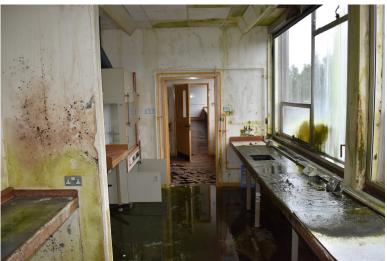
**Photograph 22** Chemistry laboratory (room A115) on first-floor, with extensive water damage visible. Photograph taken facing north-west.
