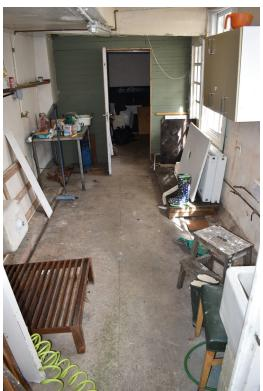
Photograph 14 Largest room in western range, showing concrete floor with drainage channels for storage of kegs. Varying ceiling heights also visible. Photograph taken facing north-west.
