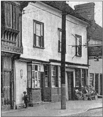
Photograph 5 North-west elevation of pub. Taken around 1935. Pargetting unclear, but appears unchanged from earlier photographs. Pub sign is new, and branding at top of elevation has been removed. Greene King Plaque has been added to east of window. Photograph taken facing west. Reproduced from www.coggeshallhistory.com.
