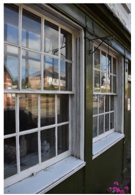
**Photograph 8** Detail of windows showing sash for pulling up shutters. Lid into recess in sill visible below windows. Photograph taken facing south.
