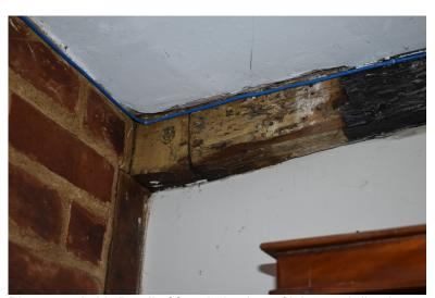
**Photograph 28** Detail of face-halved scarf joint on girding-beam between bays 1 and 2 of 17th-century main range. Photograph taken from 17th-century extension, facing west.
