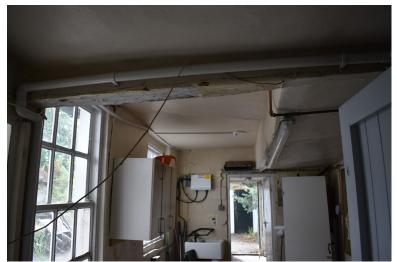
**Photograph 15** Interior of western range, showing varying ceiling heights related to 15th-century phase. Wall to left is brickbuilt, wall to right is timber. Photograph taken facing south-east.
