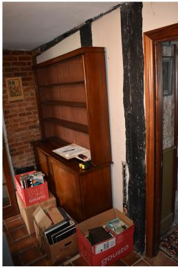
**Photograph 24** Inserted wall between 17th-century extension and main range, with large re-used studs added. Photograph taken facing west.
