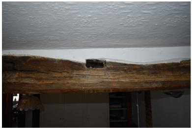
**Photograph 19** Detail of empty mortice on binding-beam in 18th-century extension. Photograph taken facing north-west.
