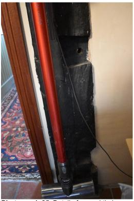
Photograph 25 Detail of reused timber with lap joints forming part of division between 17th-century extension and main range. Photograph taken facing north-west.
