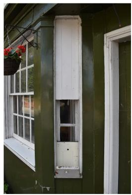
Photograph 7 Detail of sash-shutters on bay windows. Lid into recess in sill visible below window. Photograph taken facing east.
