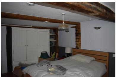
**Photograph 18** Ground-floor of 18th-century extension. Chamfered binding-beam visible in foreground, rear of 17th-century fireplace behind cupboard. Photograph taken facing north.
