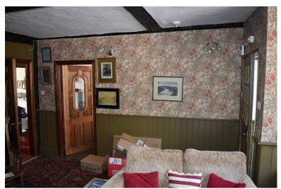
**Photograph 23** Interior of 17th-century main range, showing inserted stud wall between bays 2 and 3. The binding-beam above wall has several original pegs. Photograph taken facing west.
