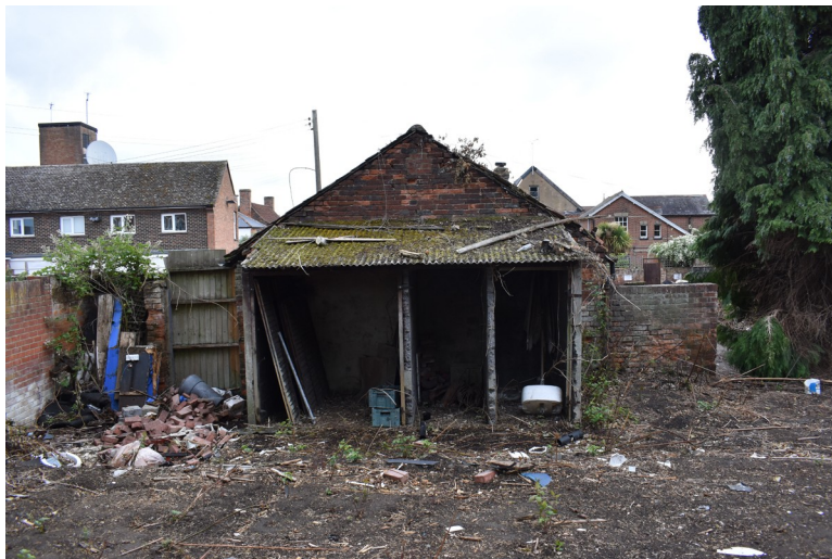
Photograph 6 South-west elevation of outbuilding, with lean-to. Photograph taken facing north-east.
