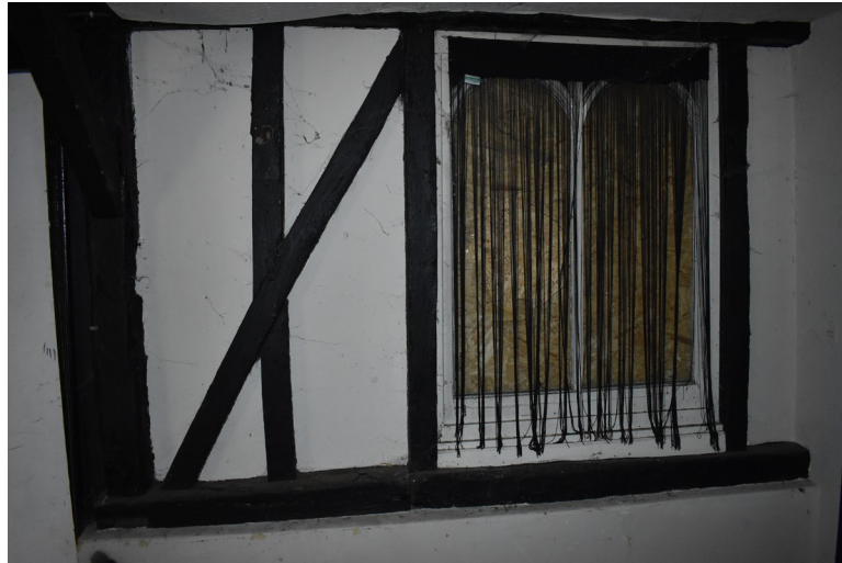
Photograph 7 Interior shot of north-west elevation of bay 4, showing fixed two-light window. Photograph taken facing north-west.
