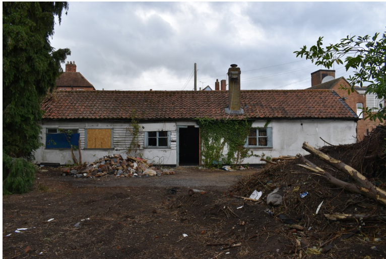
Photograph 5 South-east elevation of outbuilding. Photograph taken facing north-west.
