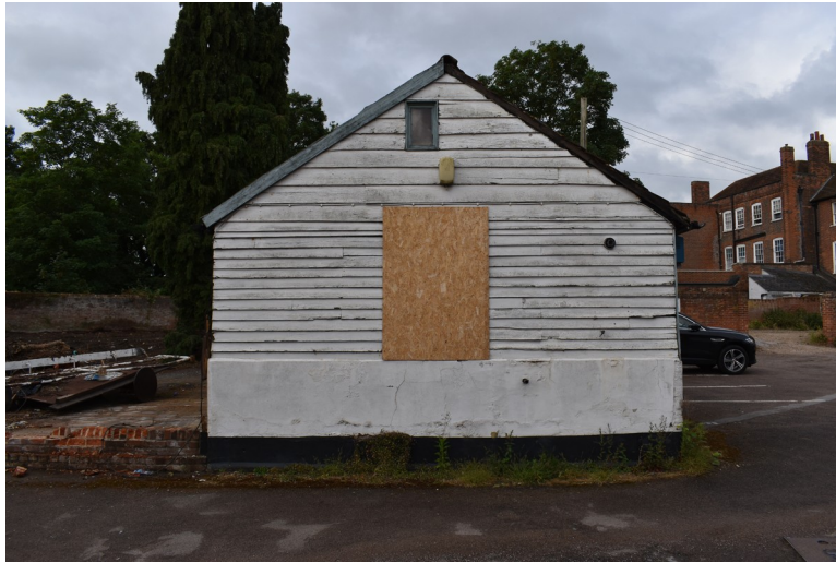
Photograph 4 North-east elevation of outbuilding. Photograph taken facing south-west.
