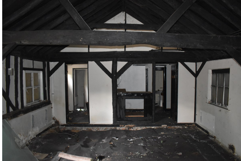
Photograph 14 The south-west elevation of bay 1, showing the original gable-end of the building. Note lack of timber-frame, suggesting prior to modern insertions this end of the building was open. Photograph taken facing south-west.
