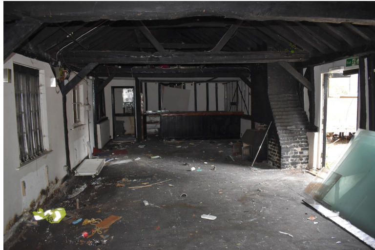
Photograph 9 Interior of outbuilding. Photograph taken from bay 1 facing north-east.
