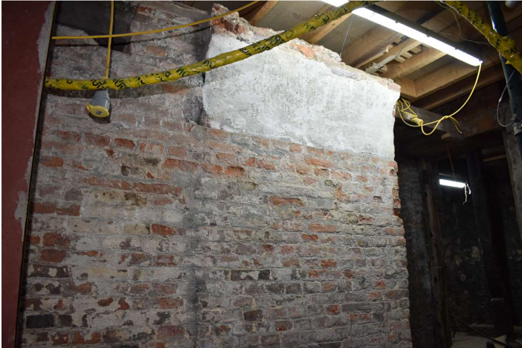
Photograph 29 Partial brick arch projecting off south of brick arch in bay 5, looking northeast.
