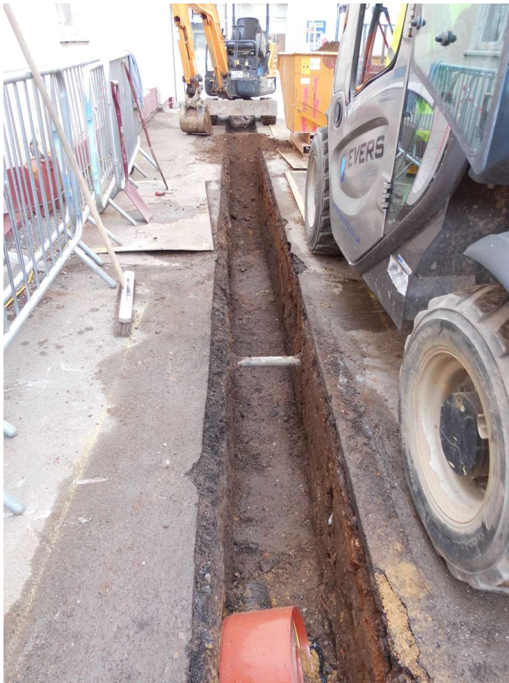
Photograph 16 The service trench in the access road, looking west.
