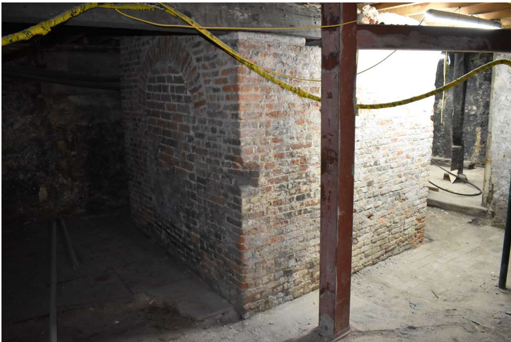
Photograph 28 Brick arch in bay 5. Blocked northern archway visible. Looking northeast.
