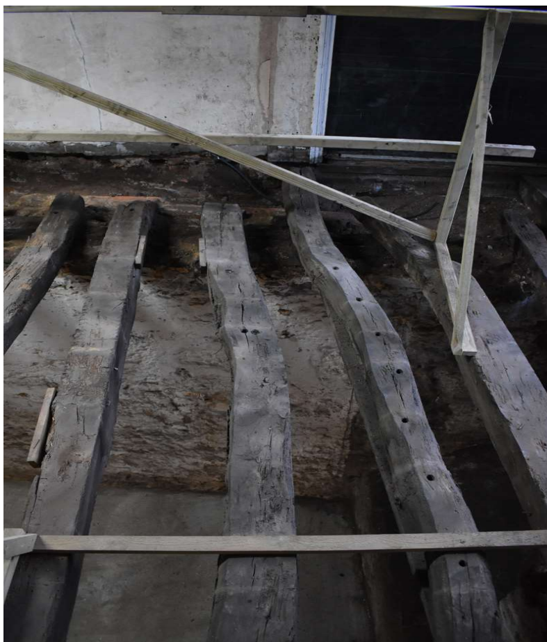
Photograph 25 Detail of sinuous joists above bay 1, looking south.
