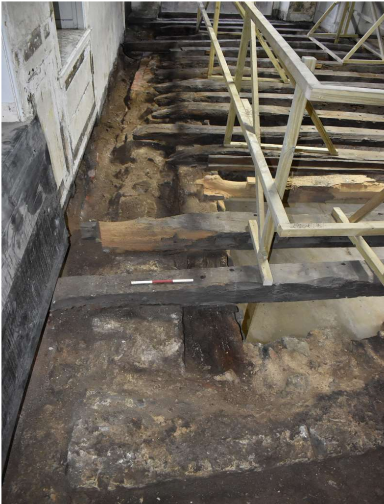
Photograph 26 Beam inserted into cellar wall supporting joists above bay 1, looking west.
