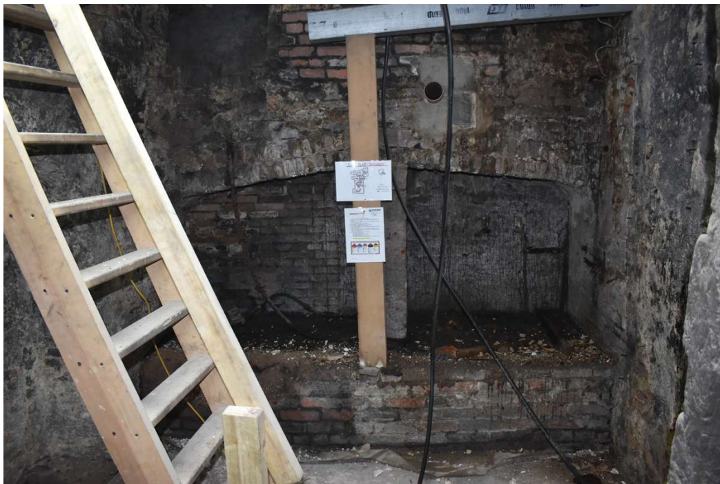
Photograph 32 Modern brickwork alcove in northern wall of bay 6, looking north.
