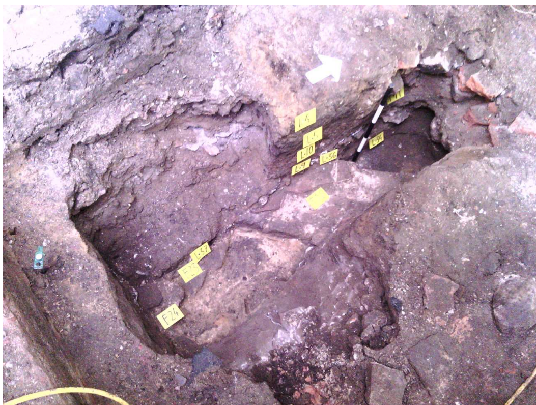
Photograph 12 Concrete sleeper pit 5 with wall foundation F22 and structural features F23 and F24, looking northwest.
