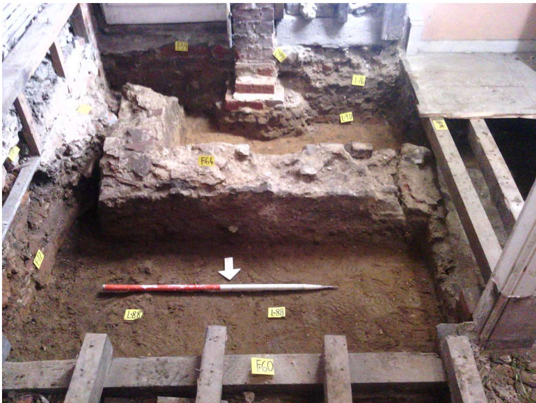
Photograph 14 The base of the lift pit showing cellar wall F64 and layers L88 and L90, looking south.
