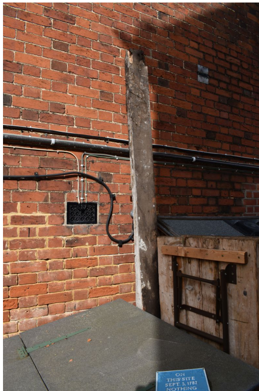
Photograph 9 Timber from demolished building, observed on site.
