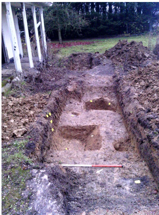
Photograph 1 T1 trench shot – looking southeast
