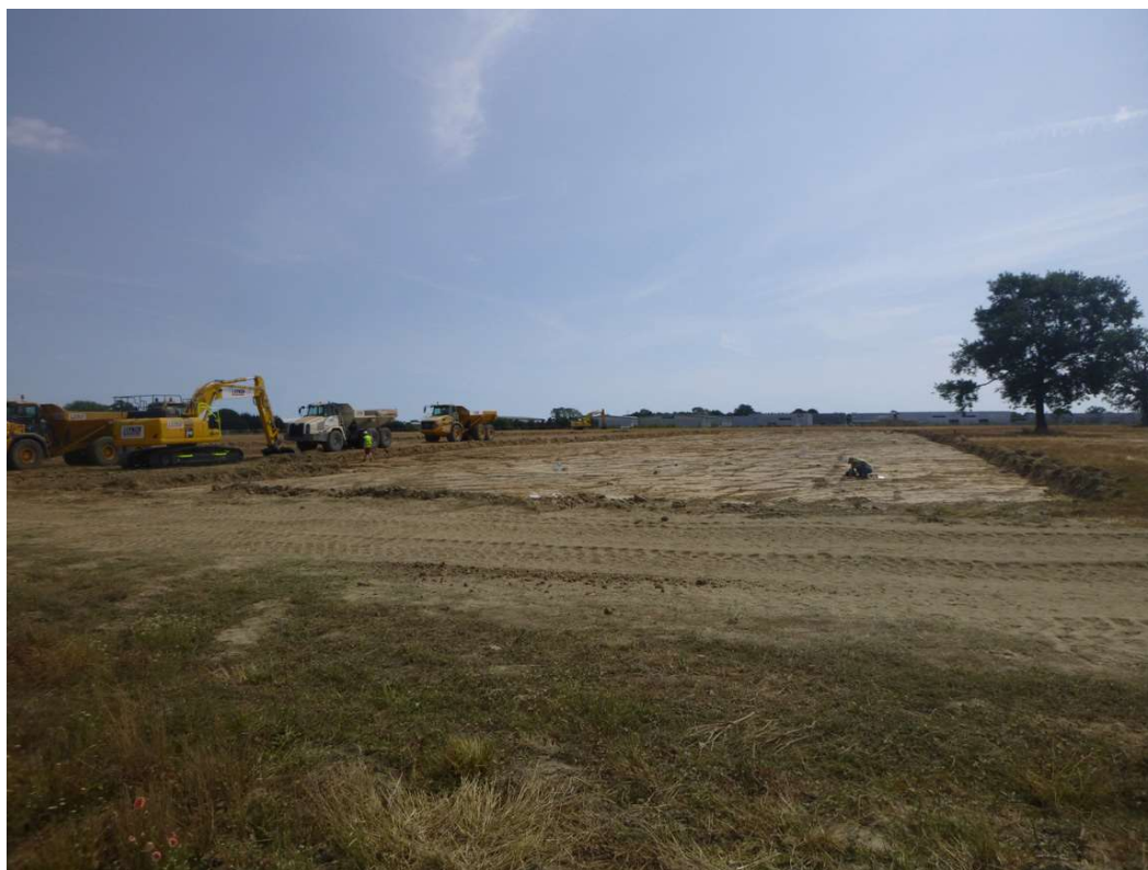
Photograph 22 Excavation: Area 1 general shot, looking south
