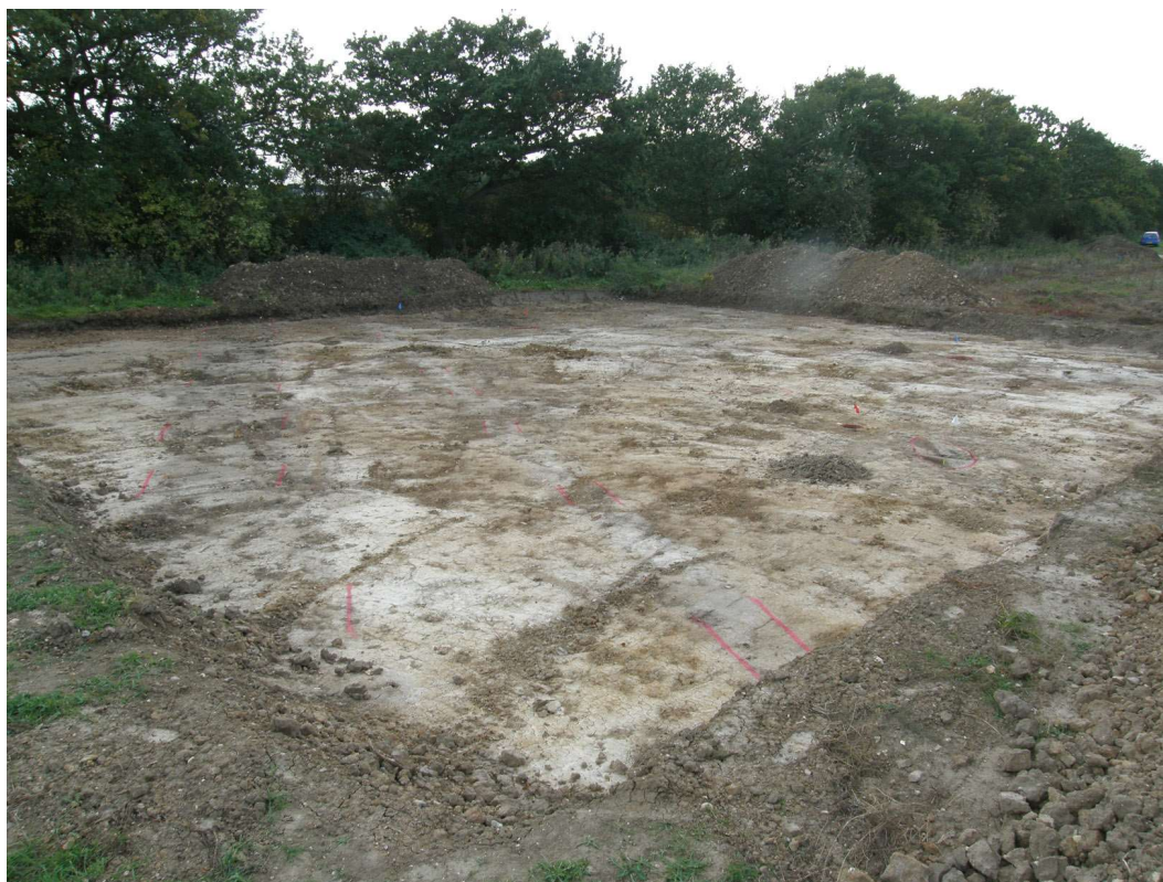
Photograph 24 Excavation: Area C general shot, looking southwest
