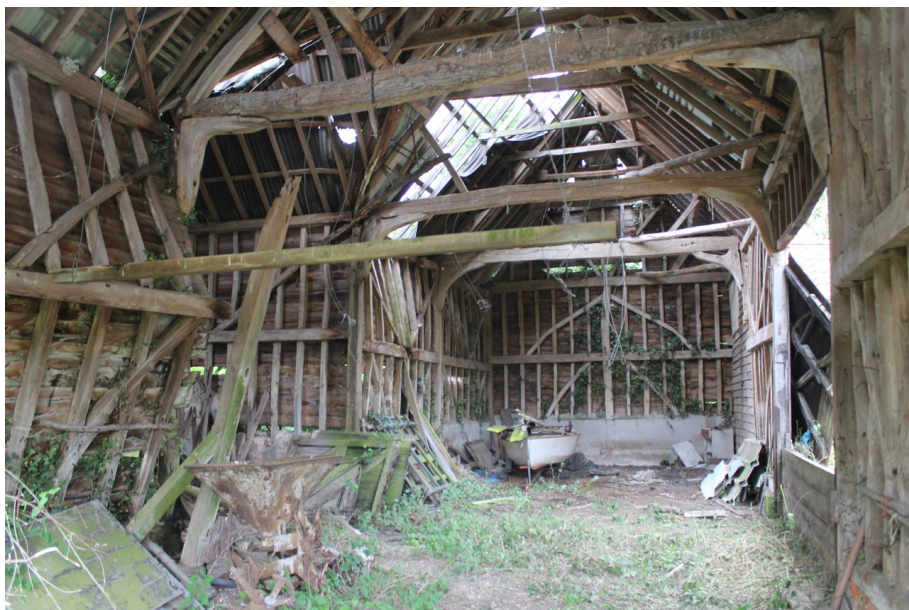
Photograph 3 Interior of threshing barn. Photograph taken facing north.
