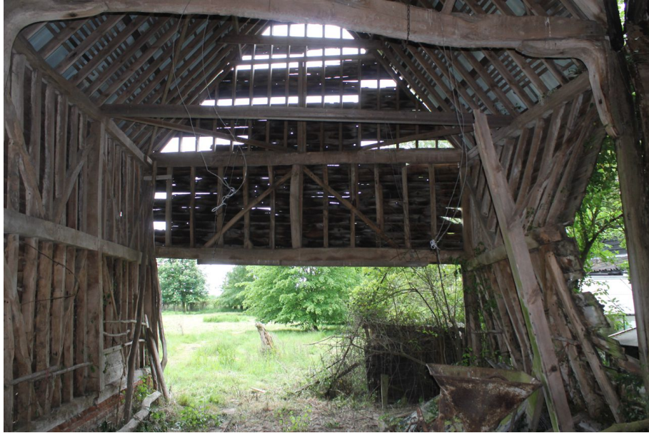
Photograph 16 South end of barn, showing bays 4 and 5. Photograph taken facing south-west.
