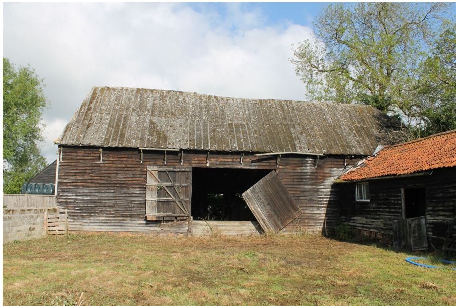
Photograph 1 South-east elevation of threshing barn. Barn doors visible in centre of elevation, brick plinth visible to left. Photograph taken facing north-west.
