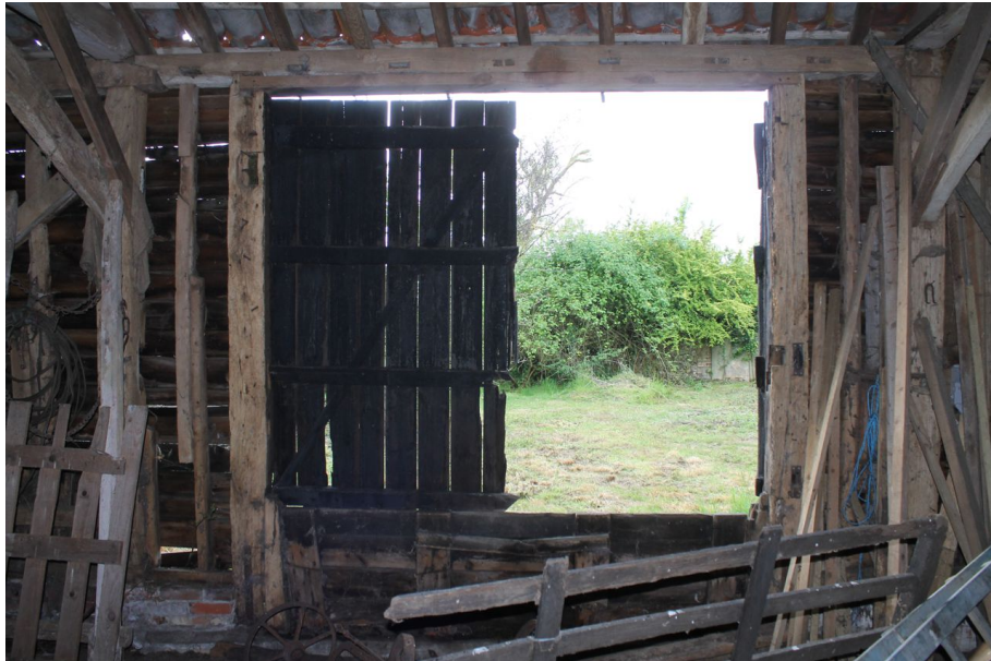
Photograph 35 Southern elevation of bay 5, showing barn door and rudimentary scarf joints on the wall-plate, with a reused timber between. Also note the reused timber used as framing for the doorway. Photograph taken facing south-west.
