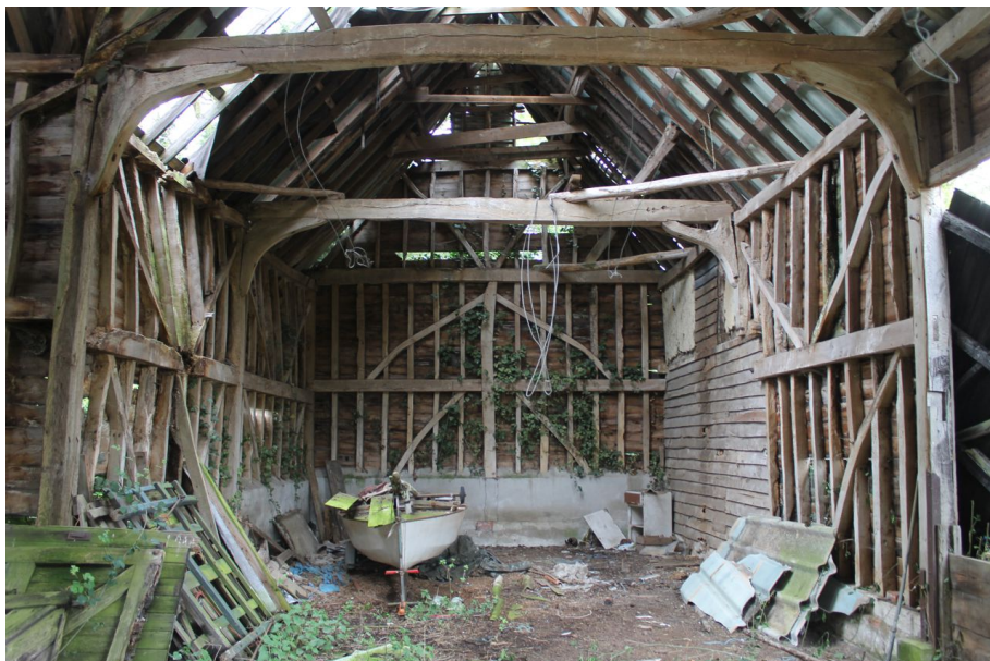
Photograph 7 North end of barn, showing bays 1 and 2. Photograph taken facing north-east.
