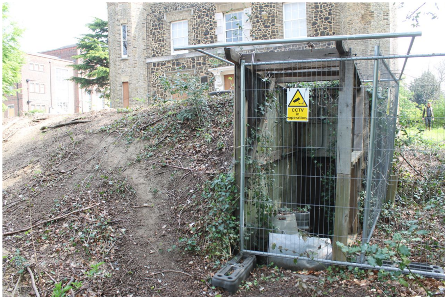
Photograph 2 Southern (blocked) entrance into air-raid shelter. Photograph taken facing north-east.
