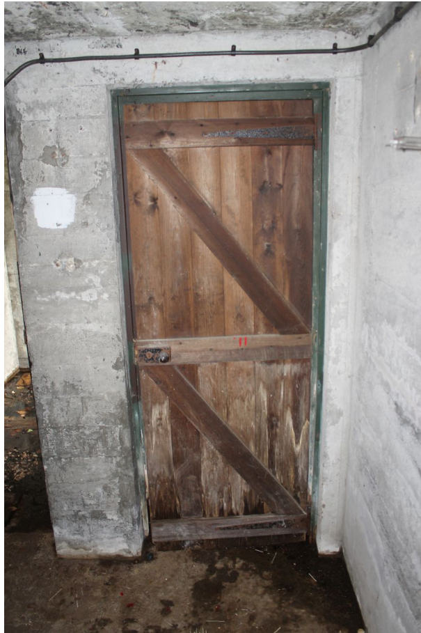
Photograph 7 Detail of northern door on interior of air-raid shelter, showing cross-battens on rear. Photograph taken facing north.
