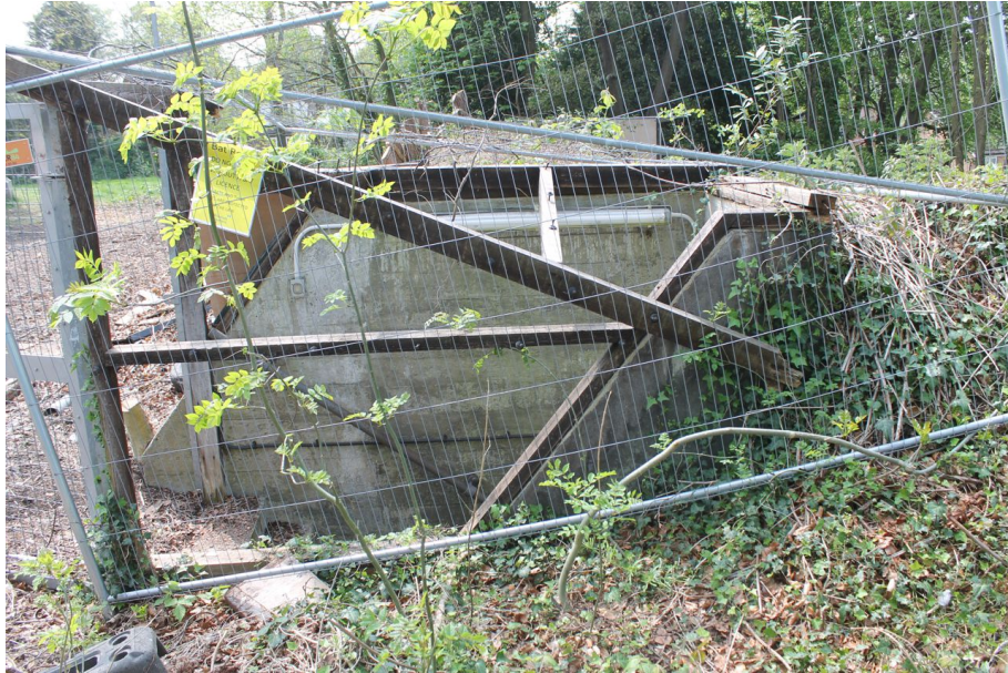
Photograph 1 Northern entrance of air-raid shelter. Photograph taken facing south-west.
