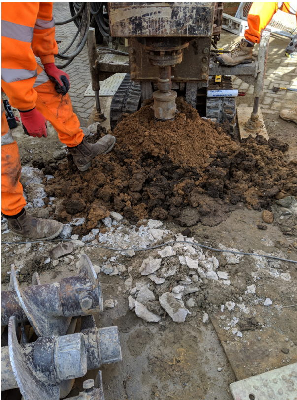
Photograph 3 Drilling of Pile 3
