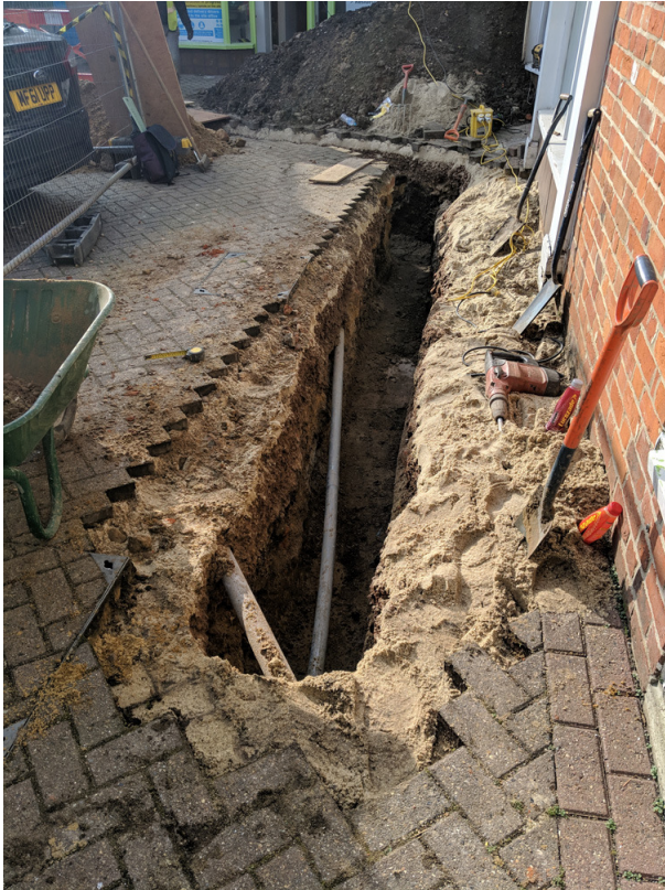
Photograph 2 Service trench, looking west
