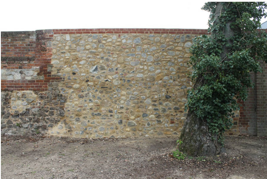
Photograph 5 West elevation of wall after repair work. Photograph taken facing east.
