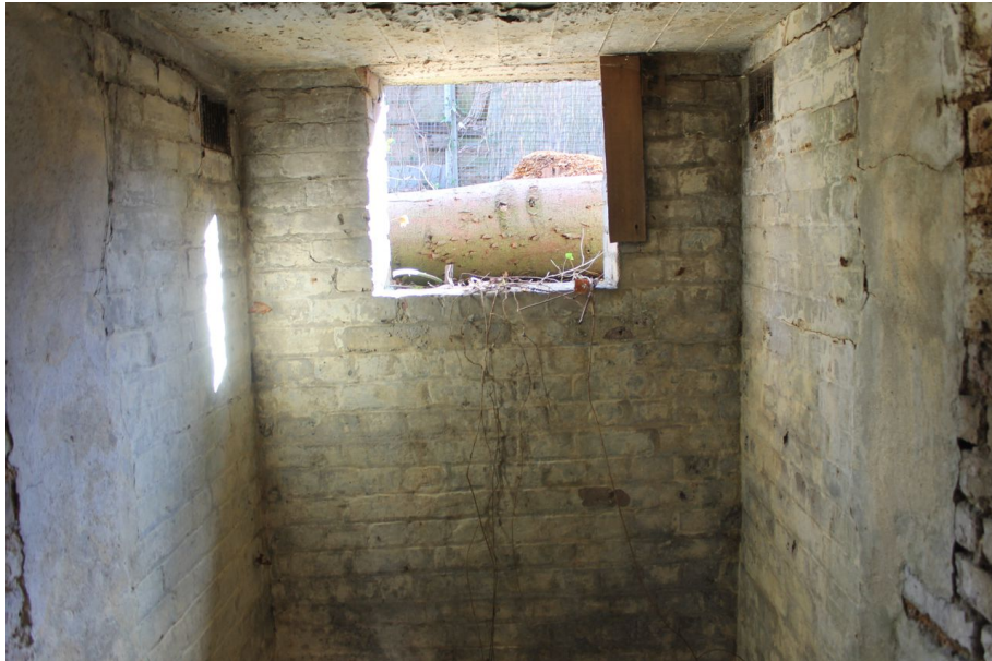
Photograph 6 Interior of air-raid shelter showing painted bricks. Photograph taken facing north-east.
