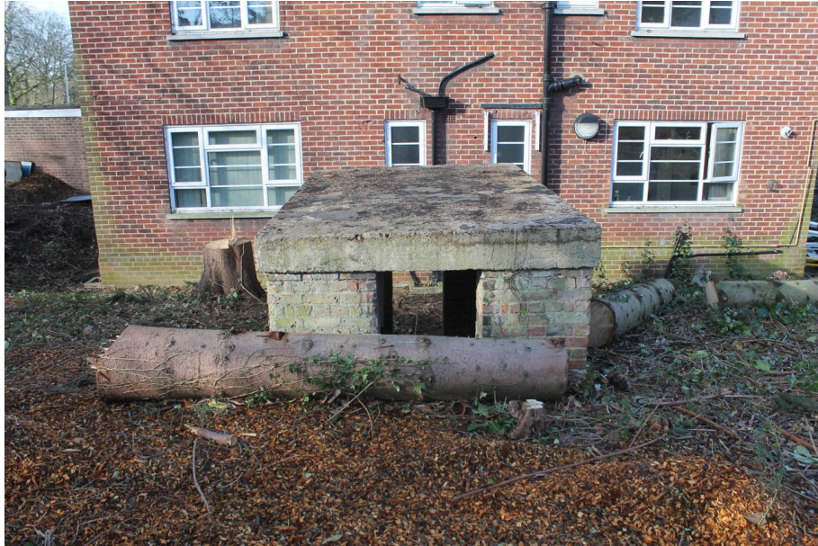
Photograph 5 North-east elevation of air-raid shelter, showing opening. Photograph taken facing south-west.
