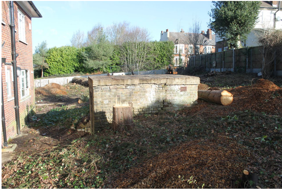
Photograph 3 South-east elevation of air-raid shelter. Photograph taken facing north-west.
