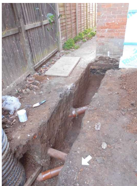
Photograph 1 Foundation trench, looking southeast
