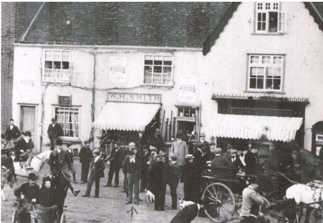
Photograph 11 The building as occupied by house furnisher W.H. Smith c 1902 (image supplied by Phil Chatfield)
