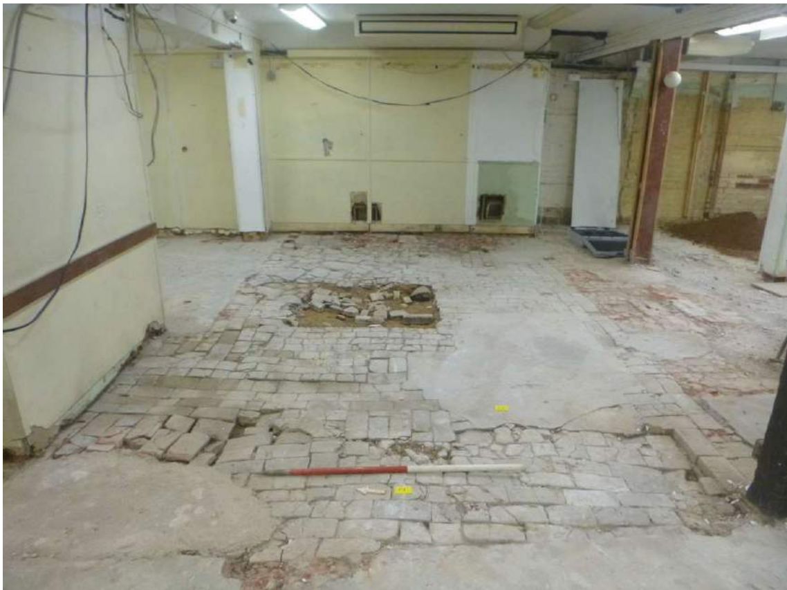
Photograph 12 Floor F1, looking east.
