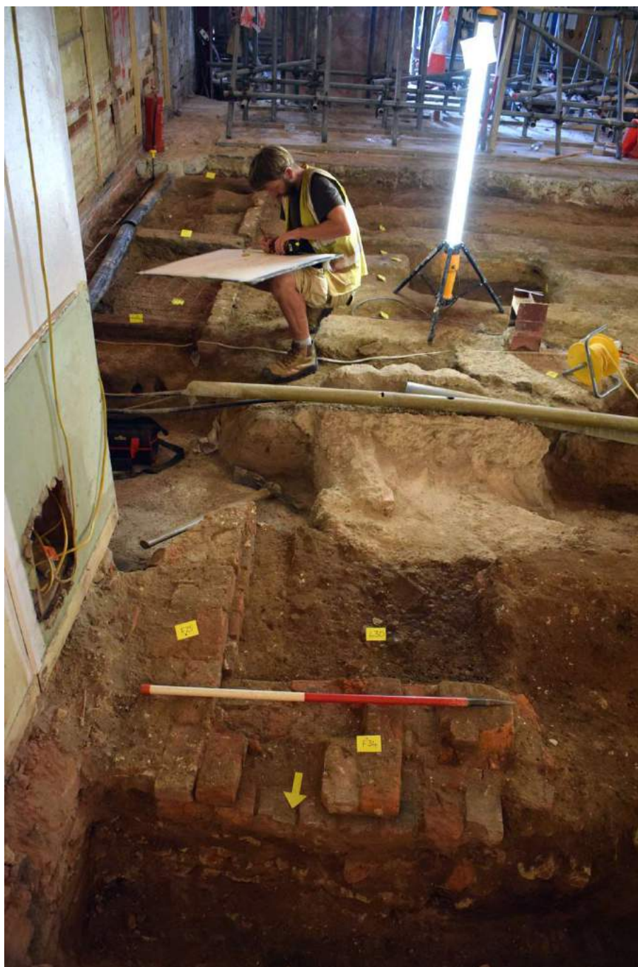
Photograph 9 Brick wall foundations F25 and F34 of the rear extension, looking south.
