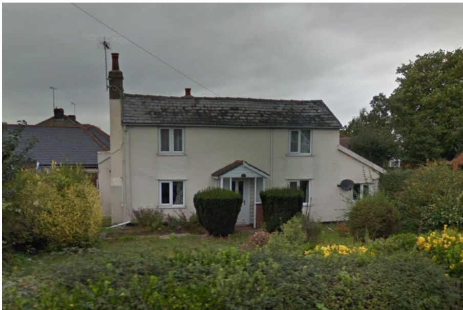
Photograph 22 South-east elevation of building prior to demolition. Porch visible, along with rendered face and modern windows of north-east extension. Photograph taken facing north-west. Copyright Google 2019, image captured September 2017.
