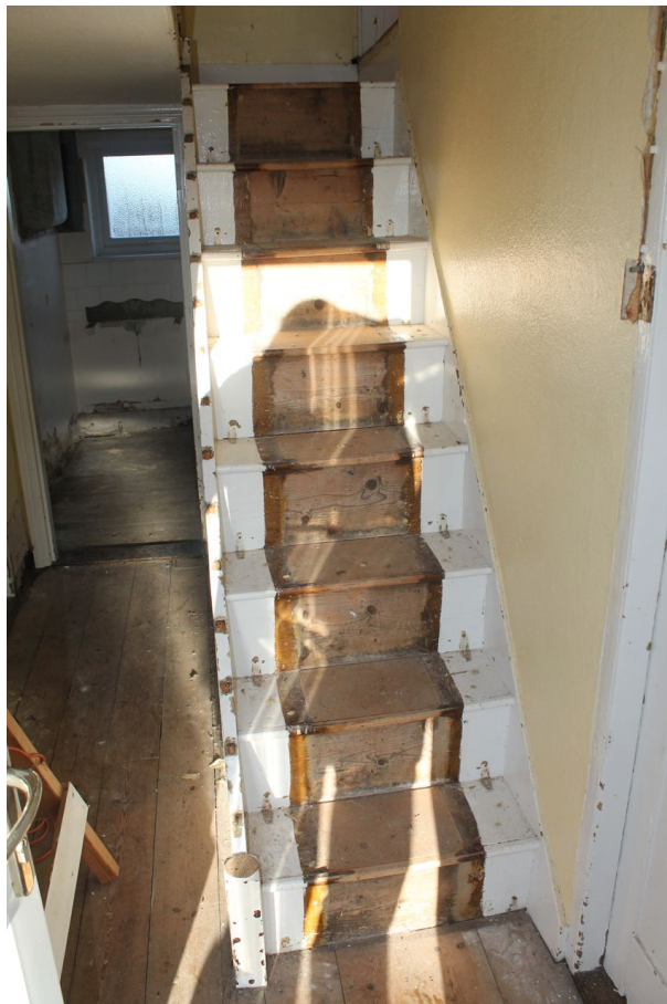
Photograph 15 Stairway in entrance hall. Photograph taken facing north-west.
