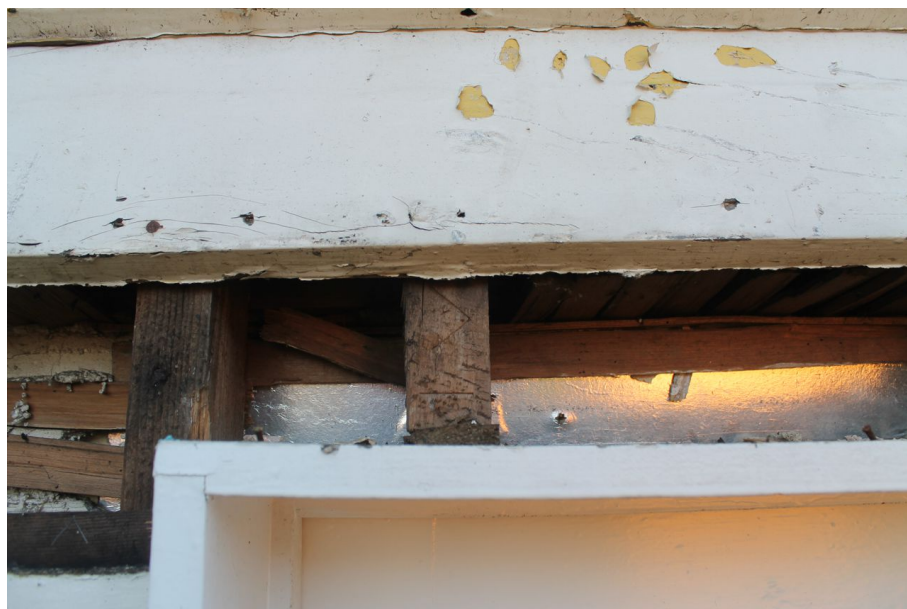
Photograph 5 Detail of chiselled carpenter's mark "IV" on stud above four-panel door on north-west elevation. Photograph taken facing south-east.
