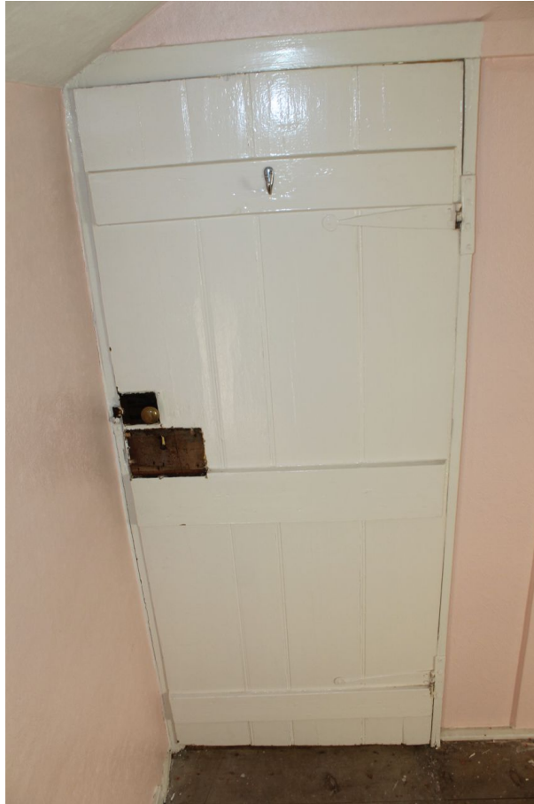
Photograph 20 Door in south-west room on first-floor. Photograph taken facing north-east.
