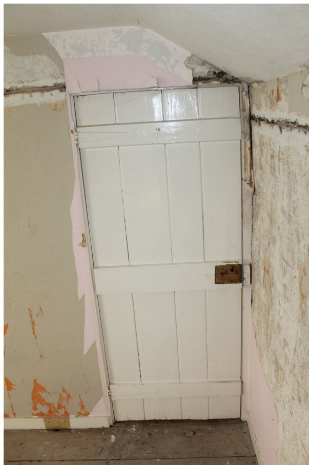
Photograph 17 Vertical-planked door in north-east room. Photograph taken facing south-west.
