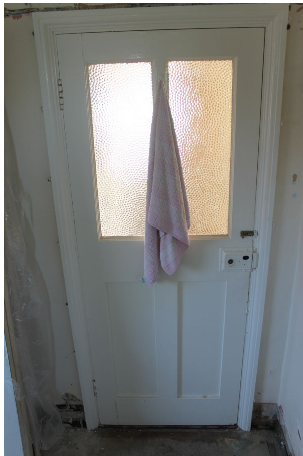
Photograph 9 Four-panel door in W.C. extension. Photograph taken facing south-east.
