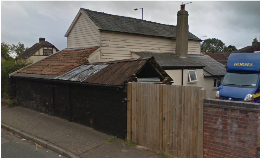
Photograph 23 North-west elevation of building prior to partial demolition. North-east extension visible as two partially(?) brick-built structures, roofed in pan-tile and corrugated metal sheeting. Apparent Flemish-bond brickwork on street frontage. Kitchen extension visible, rendered, roofed in slate and with modern? window. Photograph taken facing south. Copyright Google 2019, image captured September 2017.
