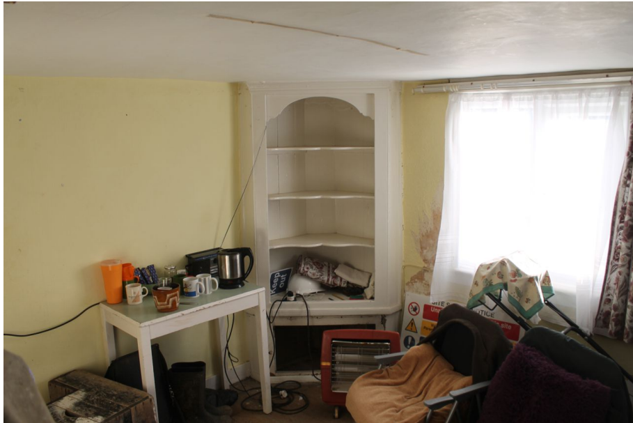
Photograph 12 Display cupboard in south-west room on ground-floor. Photograph taken facing east.
