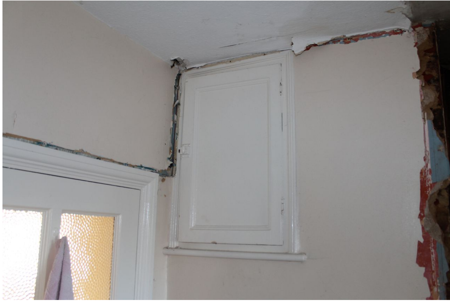
Photograph 8 Detail of cupboard in W.C. extension, built into chimney-stack. Photograph taken facing south.
