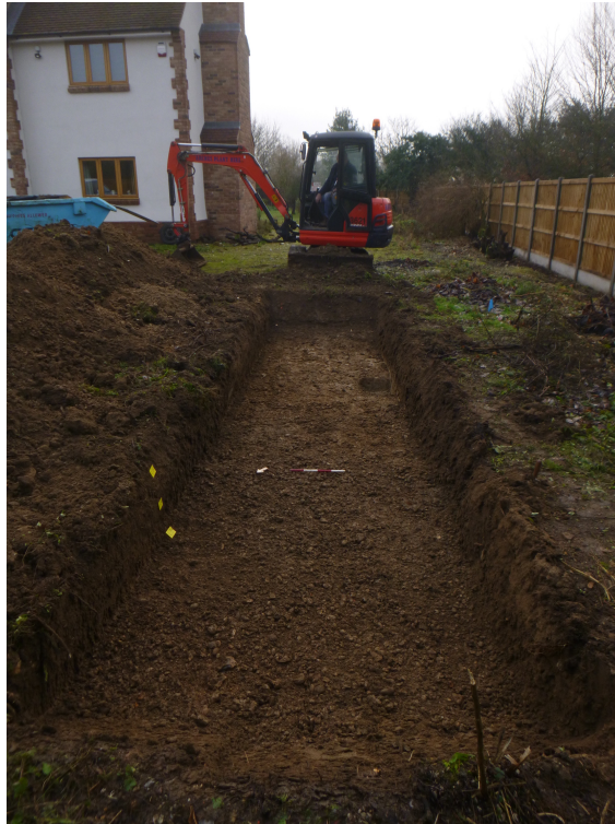
Photograph 1 Trench shot, looking south southeast
