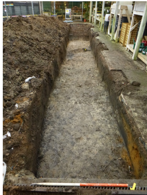
Photograph 2 T3 trench shot – looking SSE
