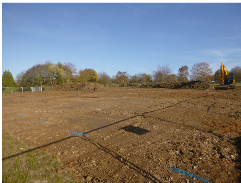
Photograph 1 Machine strip of temporary car park 1.
