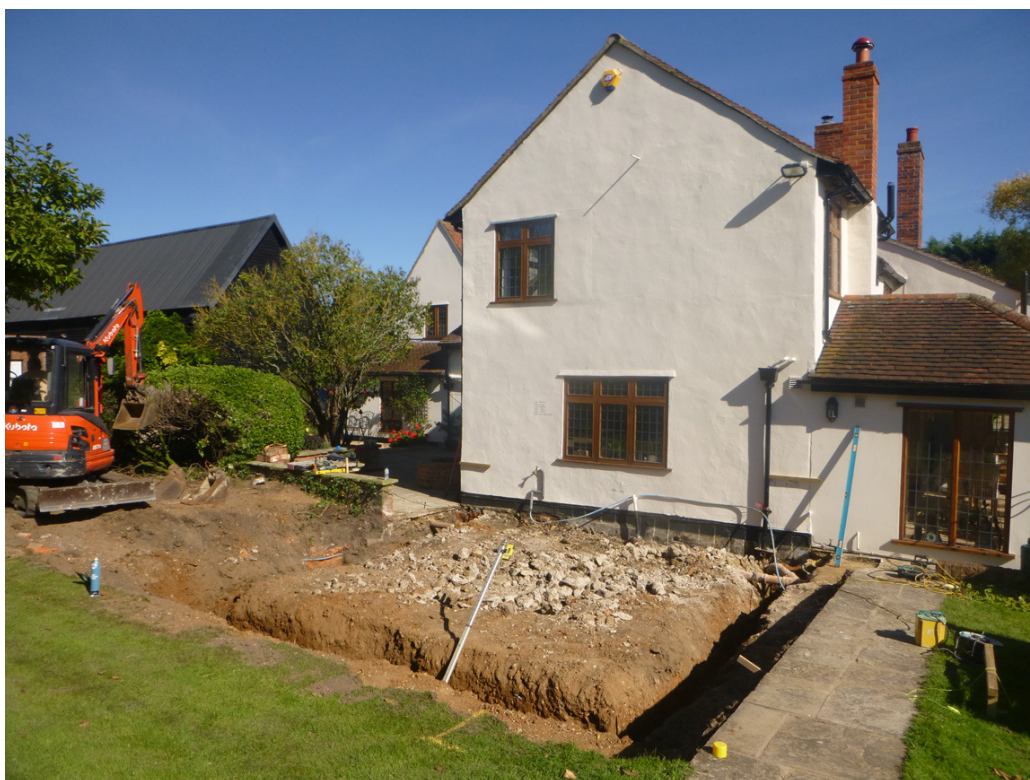
Photograph 1 Area of level reduction and foundation trenches, looking northeast
