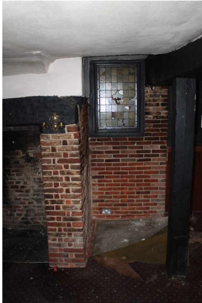
Photograph 16 North-east ground-floor wall to Structure A, showing inserted brickwork and stained-glass window. Photograph taken facing north-east.
