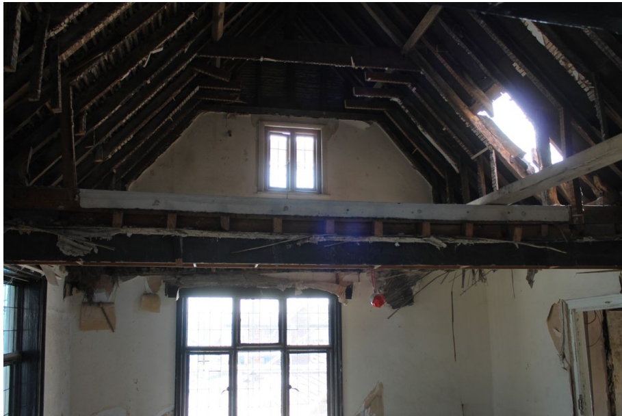
Photograph 56 Southern-most tie-beam in Structure C, showing secondary modern timber attached to its upper face for reinforcement. Photograph taken facing south-west.
