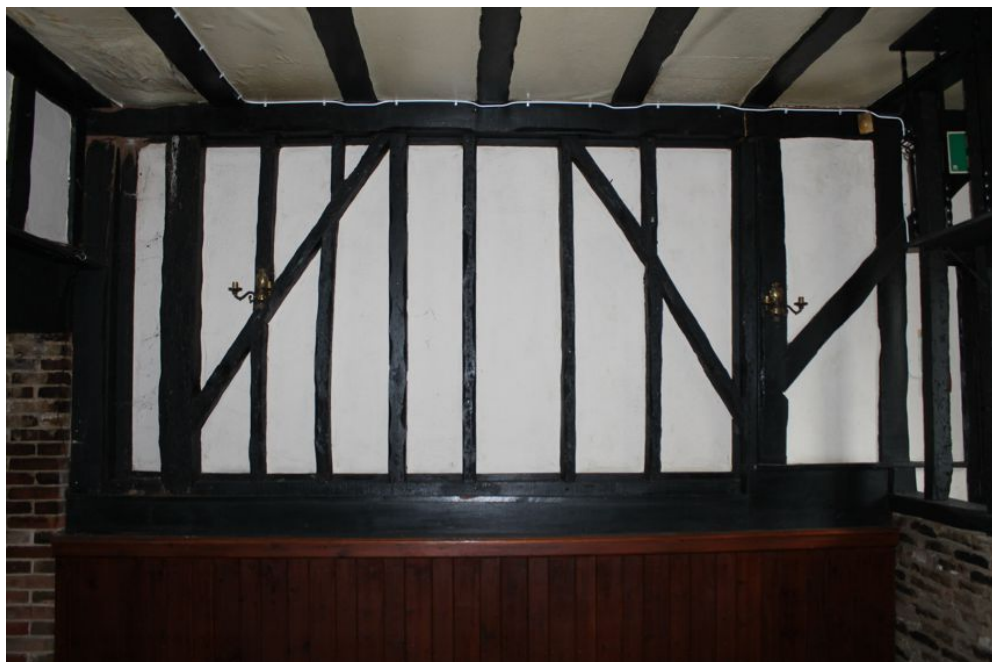
Photograph 40 Stud-work on north-east elevation of Structure F, including some re-used timbers. Photograph taken facing north-east.
