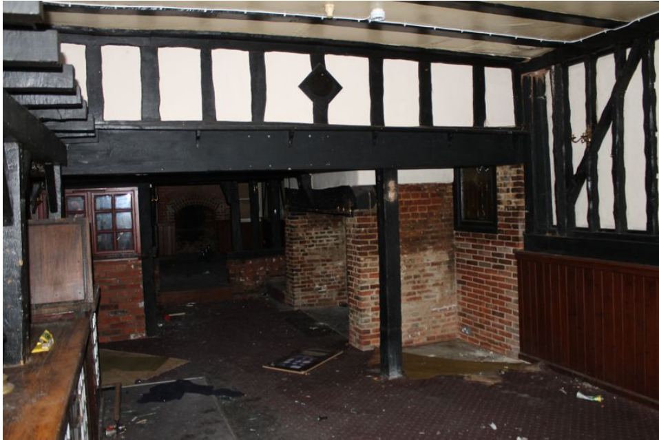
Photograph 13 South-east elevation of Structure A from interior of Structure F. Inserted beam and post visible. Photograph taken facing north-west.
