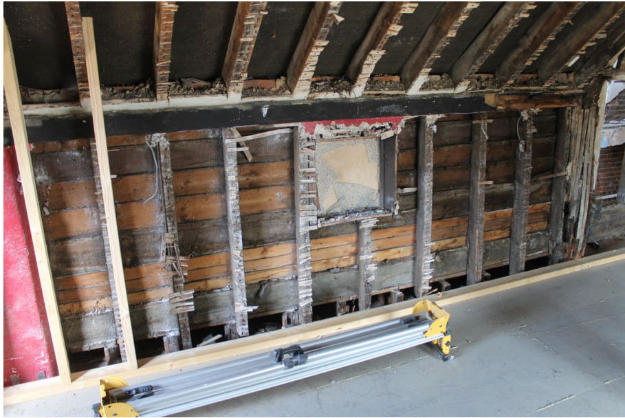
Photograph 51 Exposed machine-cut timber-frame of Structure B on north-east elevation, including inserted window. Photograph taken facing east.
