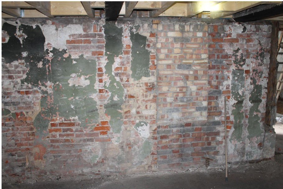
Photograph 52 Exposed brick wall on ground-floor of Structure B, north-east elevation. Photograph taken facing north-east.
