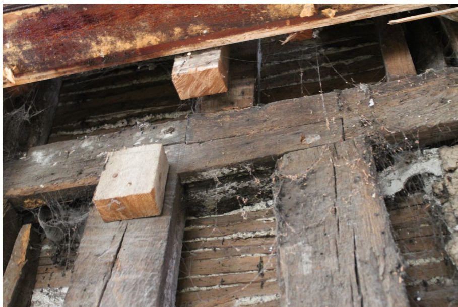
Photograph 46 Detail of scarf joint on south-east girding-beam of Structure A. Photograph taken facing north-west.
