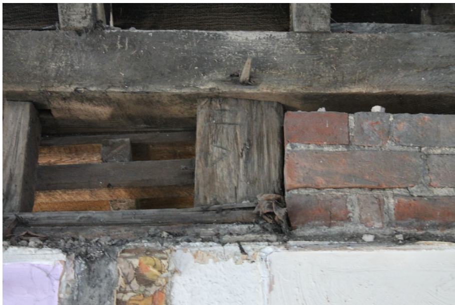
Photograph 57 Detail of carpenter's mark "VII" on stud/storey-post in north-west elevation of Structure C. Photograph taken facing north-west.
