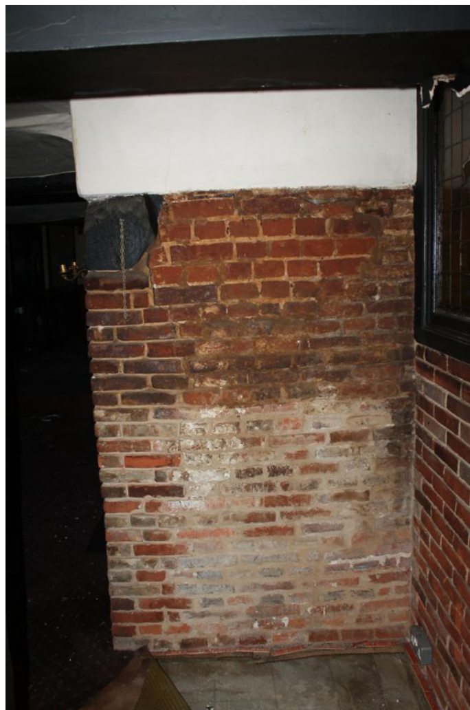
Photograph 15 South-east side of fireplace, showing rebuilt areas compared to original brickwork. Photograph taken facing north-west.
