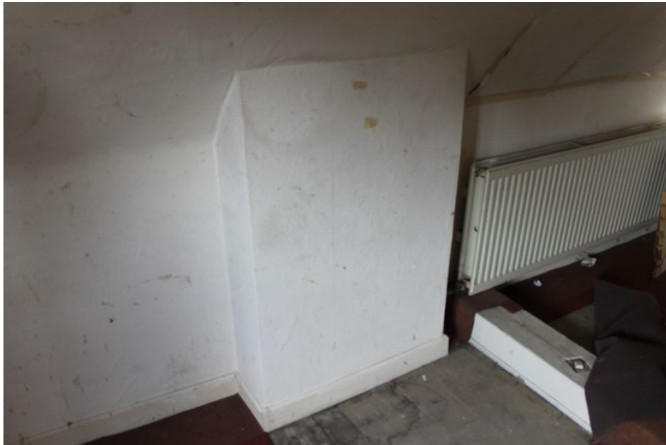
Photograph 33 Blocked fireplace and exposed tie-beam on second-floor of Structure C. Photograph taken facing north.
