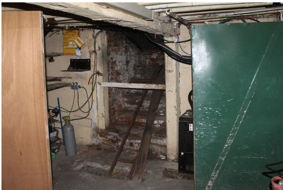
Photograph 30 Cellar below Structure C, showing barrel chute from pavement. Photograph taken facing east.
