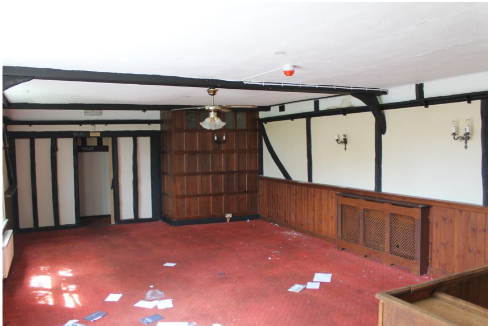
Photograph 32 ground-floor of Structure C. Photograph taken facing west.
