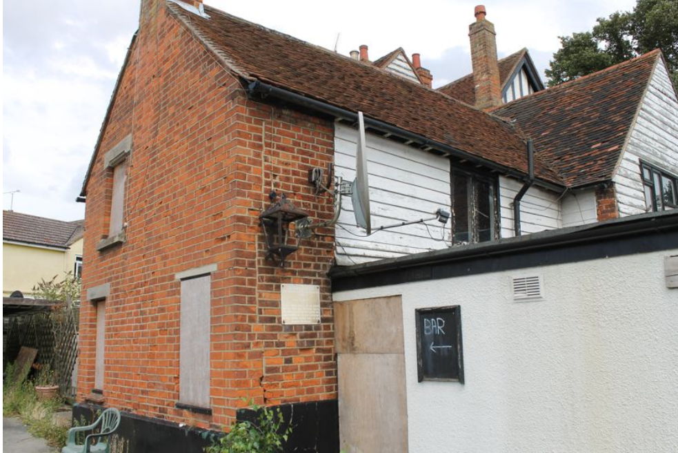
Photograph 9 North-west and south-west elevations of Structure B, showing mismatched brickwork adjacent to timber-frame. Photograph taken facing east.
