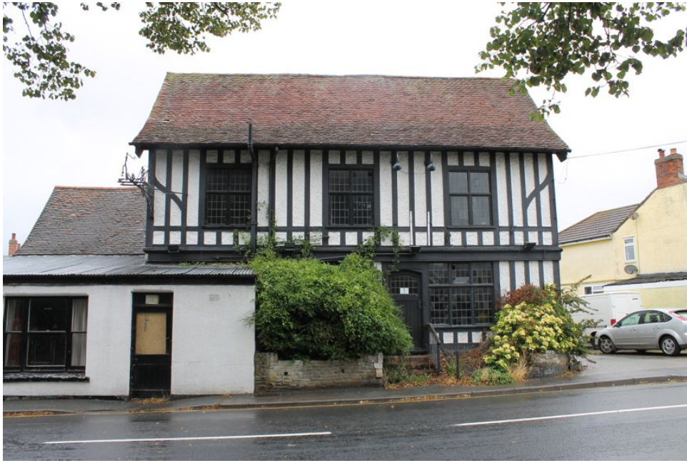
Photograph 11 South-east elevation of Structure C. Photograph taken facing south-west.
