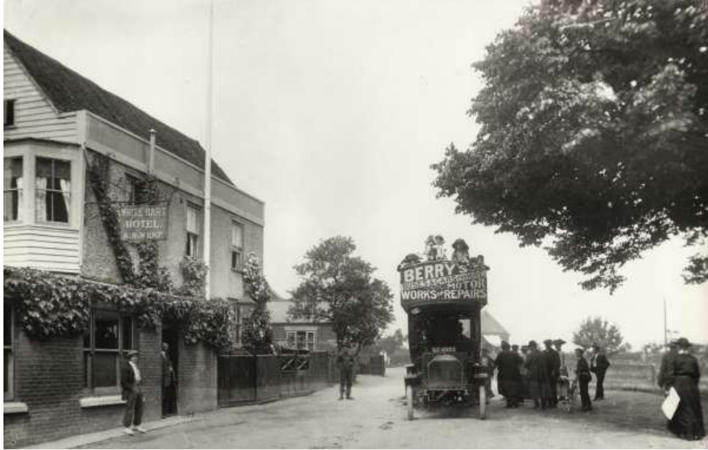
Photograph 3 1910 photo showing the south-eastern elevation of Structures C and F. Same appearance as in Photograph 2, above, but this angle also shows the edge of an oriel window (which is no longer extant) on the south-west elevation of Structure C. The original bus terminus from Colchester was located outside the White Hart (as evidenced by the bus in this photo). Taken from www.merseamuseum.org.uk .
