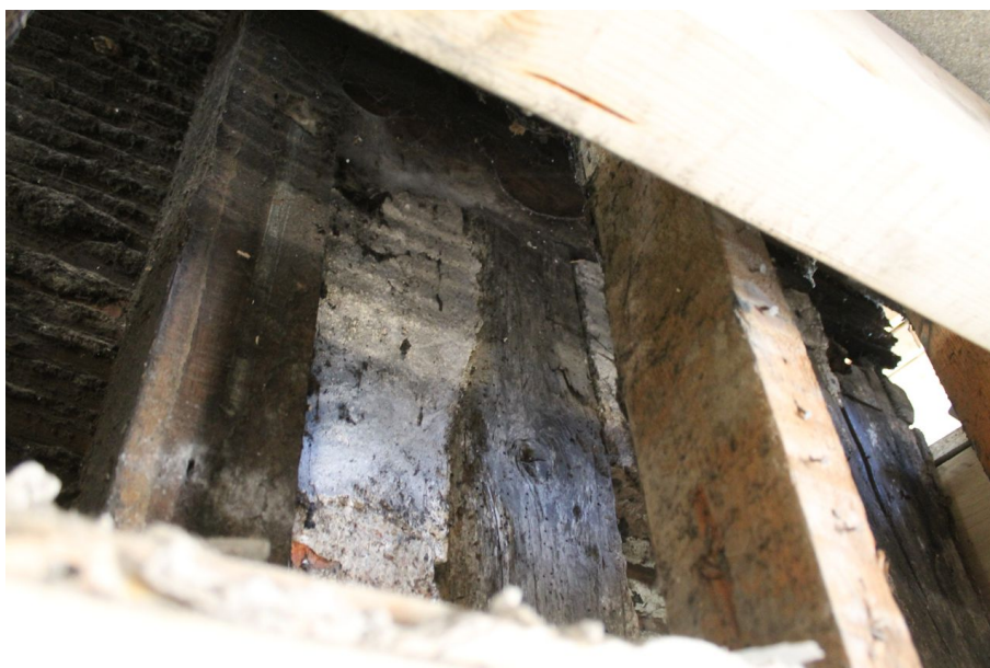
Photograph 50 Timber and plaster behind chimney stack in Structure A. Photograph taken facing west.
