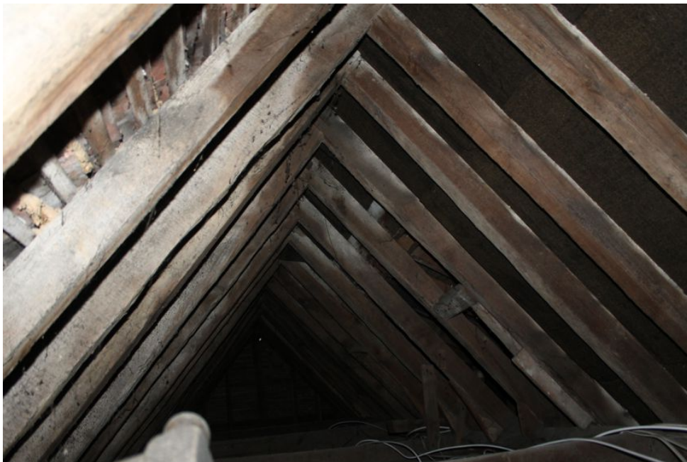
Photograph 34 Roof structure of Structure C. Photograph taken facing south-west.
