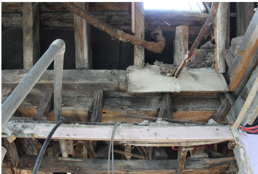
Photograph 60 Detail of scarf joint on north-west wall plate of Structure C. Photograph taken facing north-west.
