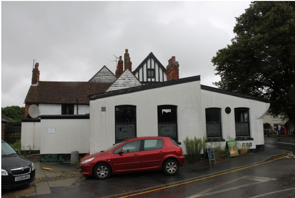
Photograph 10 South-west elevation of White Hart. Photograph taken facing north-east.
