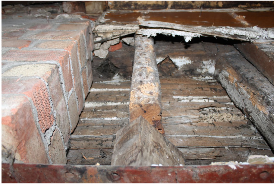
Photograph 47 Detail of diamond mullion mortices on underside of Structure A's south-east girding-beam. Photograph taken facing north-west.
