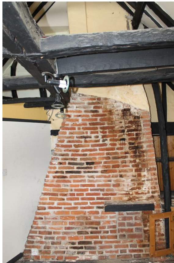
Photograph 19 Chimney stack in north-east first-floor wall of Structure A. Photograph taken facing north-east.
