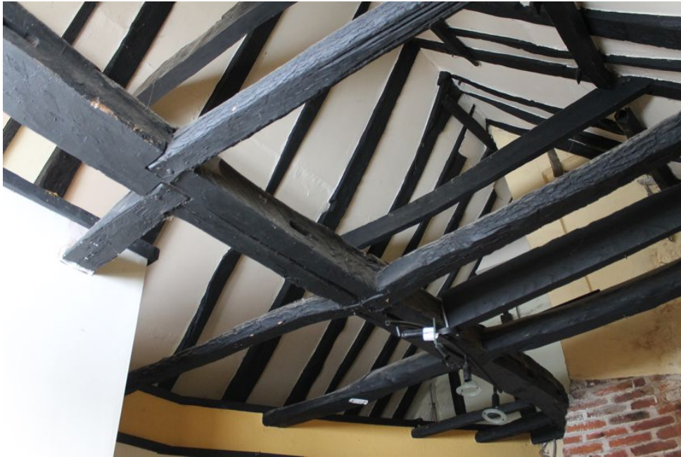
Photograph 20 Roof structure of Structure A, showing collar-purlin and braces. Photograph taken facing north.
