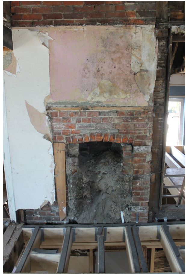
Photograph 54 Exposed fireplace in first-floor of Structure C. Photograph taken facing north-west.
