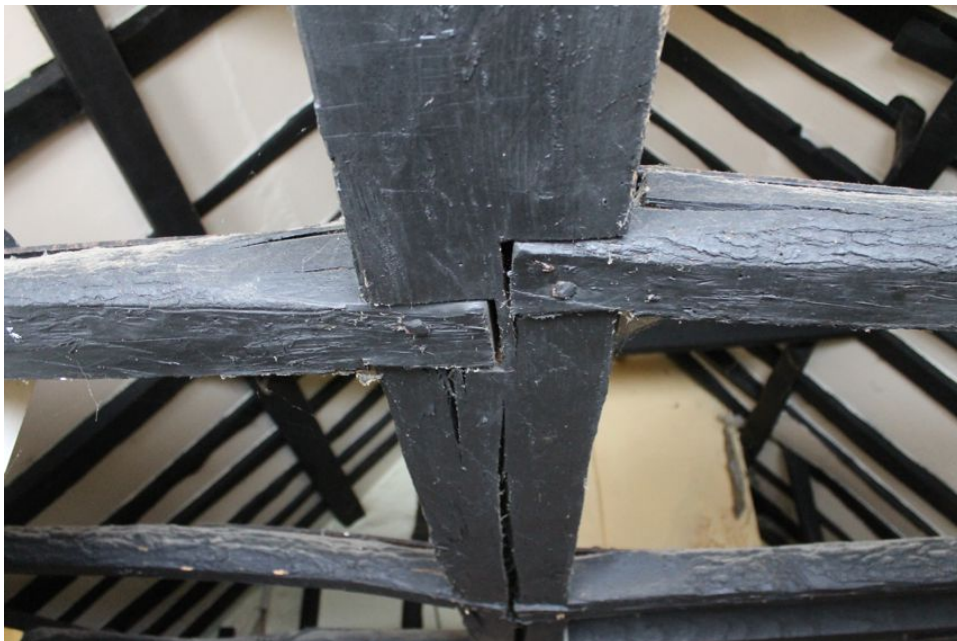
Photograph 21 Detail of underside of collar-purlin, showing joggled lap-joints. Photograph taken facing north-east.
