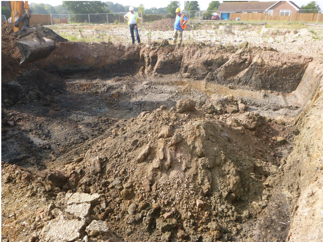
Photograph 2 Excavation of the contaminated backfill from the pond.
