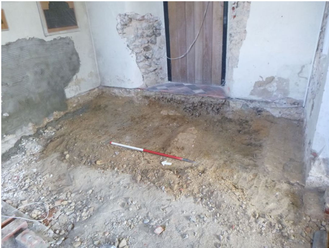
Photograph 2 Detail of east of Chapel floor after cleaning. Original lime mortar floor (F2) visible in corners. Brick pads (F1) visible in centre. Photograph taken facing east.
