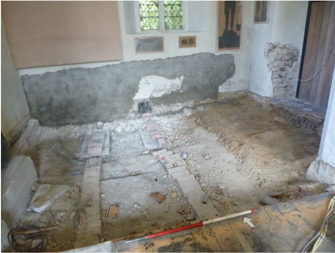
Photograph 1 Interior of Chapel after floor removed. Brick and concrete supports (F1) visible to left. Photograph taken facing north-east.
