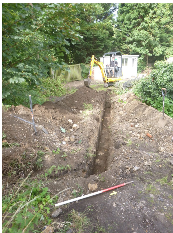
Photograph 2 Trench for water pipe under excavation. Photograph taken facing north-west.
