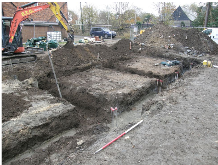
Photograph 1 South-west corner of foundation trench during excavation. Photograph taken facing east.
