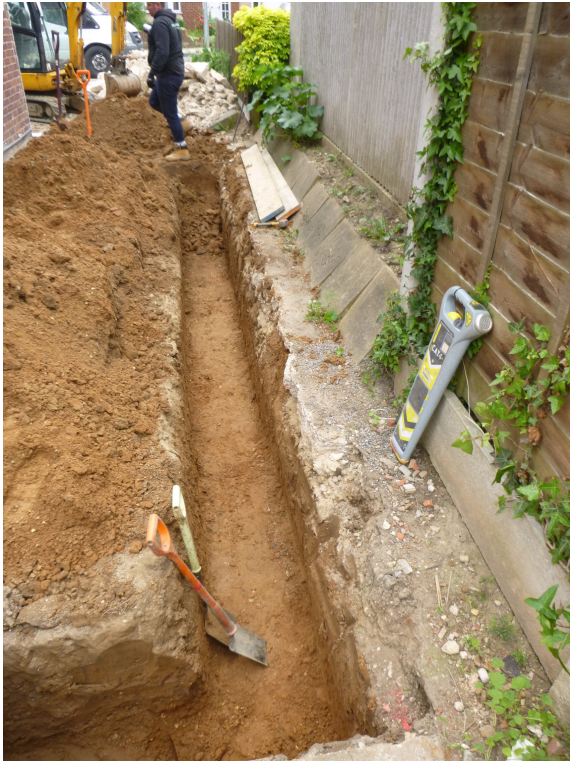
Photograph 1 Foundation trenches, looking south
