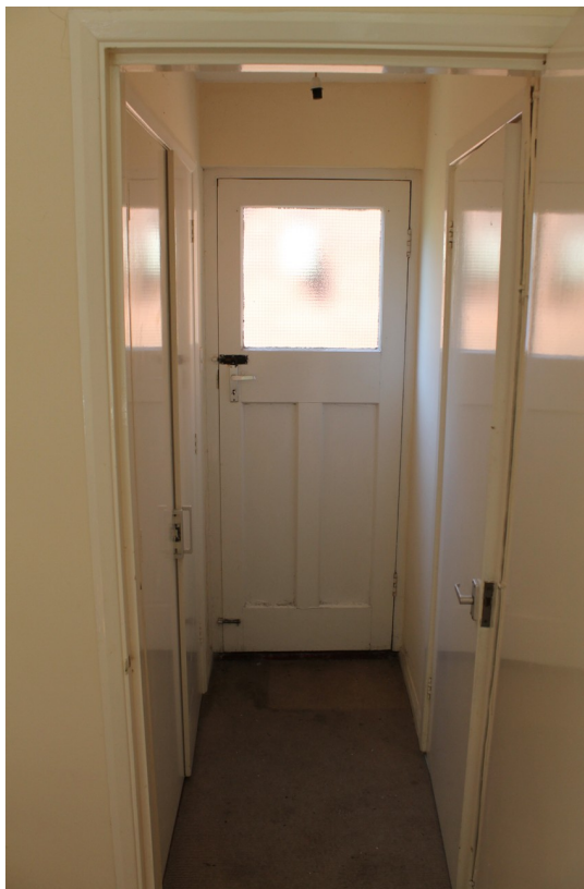
Photograph 23 1962 bathroom extension to No.7 Winnocks, with storage cupboard to the left and bathroom on the right – view north-west.
