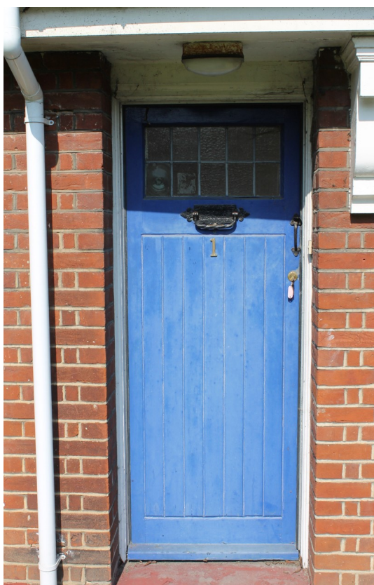
Photograph 4 Original door to No.1 Winnocks – view north-west.
