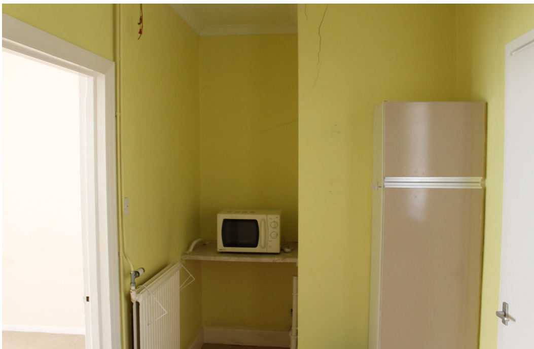
Photograph 16 Kitchen of No.3 Winnocks: the original coal store was located to the left, now a handy nook for a microwave. The pantry has been blocked off from the kitchen and turned into the WC for the 1962 bathroom extension - view south.
