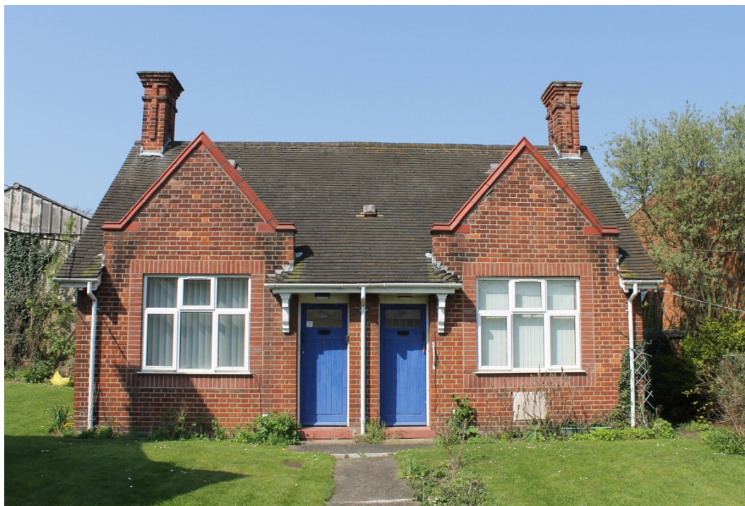
Photograph 3 East elevation of Nos.3-4 Winnocks: the windows are replacement UPVC frames set into a brick surround. The doors appear to be original – view west.
