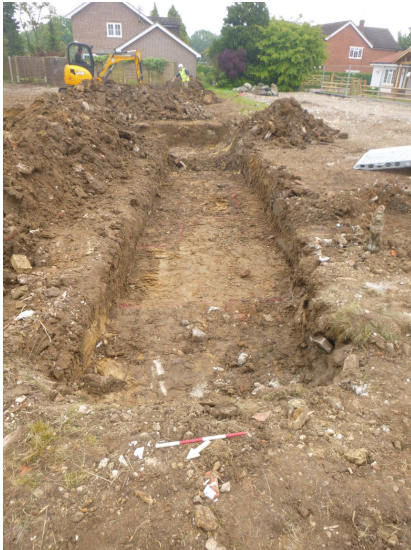
Photograph 1 Trench T1a, looking SE
