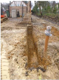
**Photograph 2** Foundation trenching in southern part of plot 2
