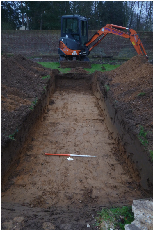
Photograph 1 Trench T1, looking E
