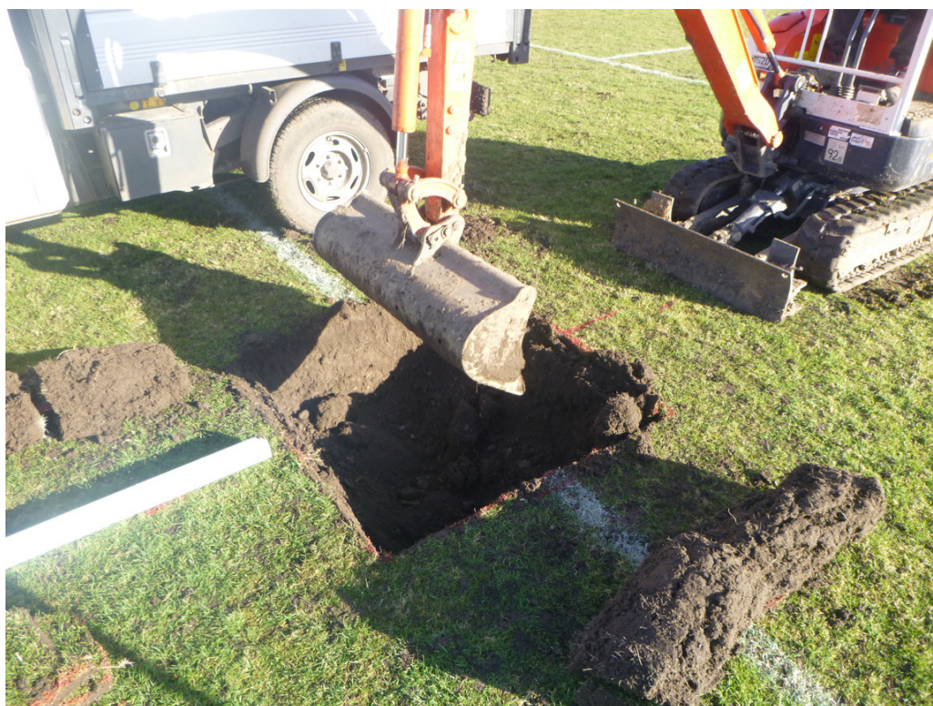
Photograph 1 Foundation post 1 under excavation, looking northeast
