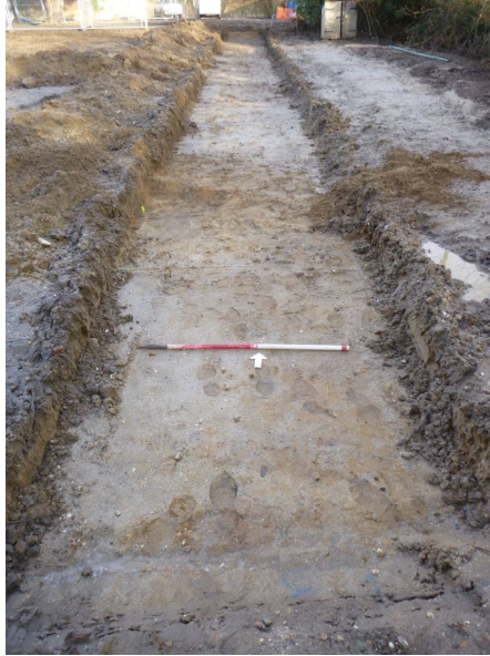
Photograph 4 T3 trench shot – looking north
