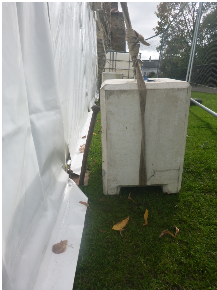
Photograph 8 Pegs securing marquees, looking S
