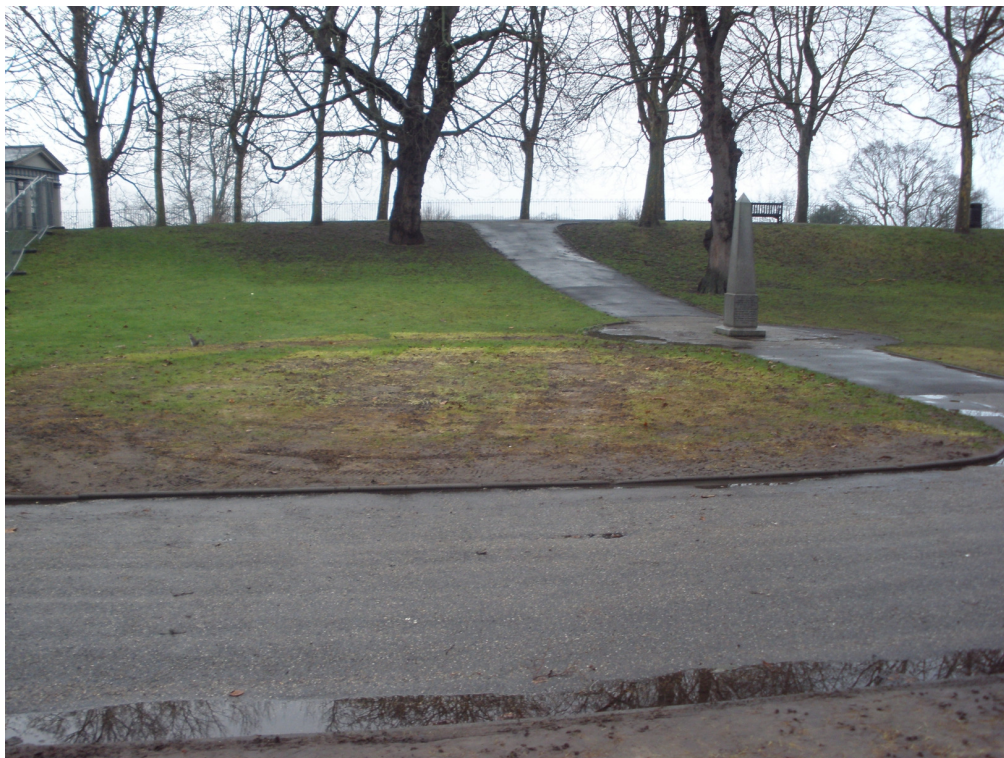
Photograph 10 Damage to grass north of the Castle post-events, looking N
