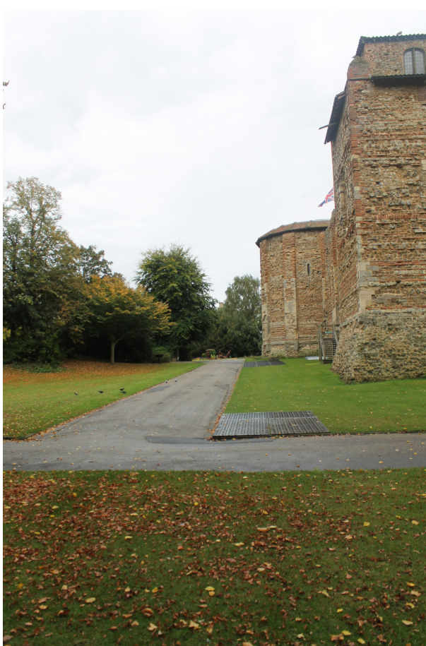
Photograph 2 East side of Castle before the events, looking S
