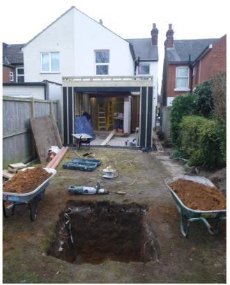
Photograph 3 Excavation of soakaway, looking SW.
