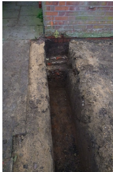
Photograph 1 Trench shot – looking south-east
