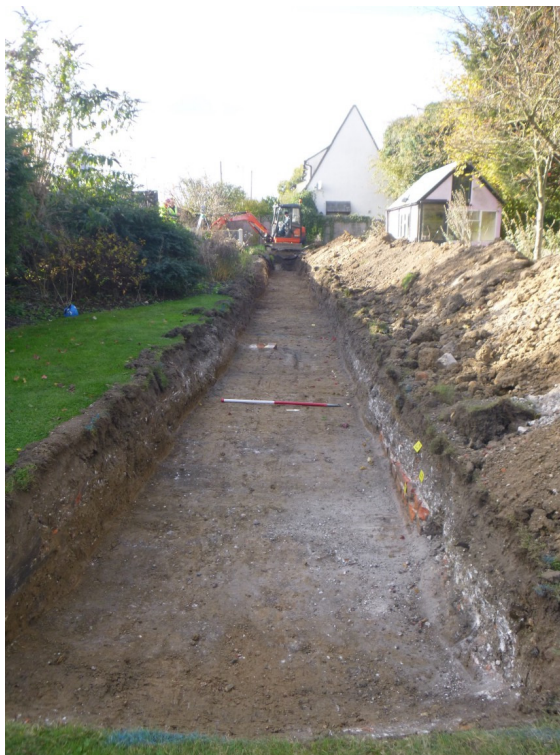
Photograph 1 T1 trench shot – looking west
