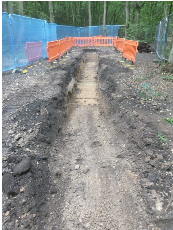
Photograph 1 Last section of trench – looking north
