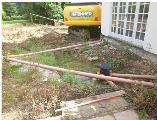
Photograph 1 Modern ditch - looking north northeast
