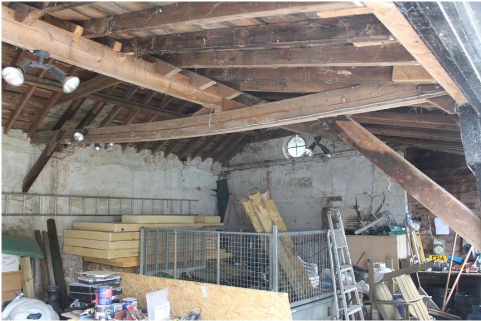
Photograph 7 Interior of outbuilding and outshot - looking north.
