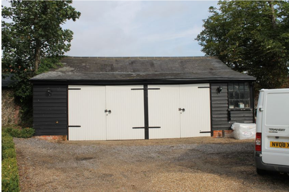
Photograph 3 Southeast elevation of outshot, showing large double doors – looking northwest.
