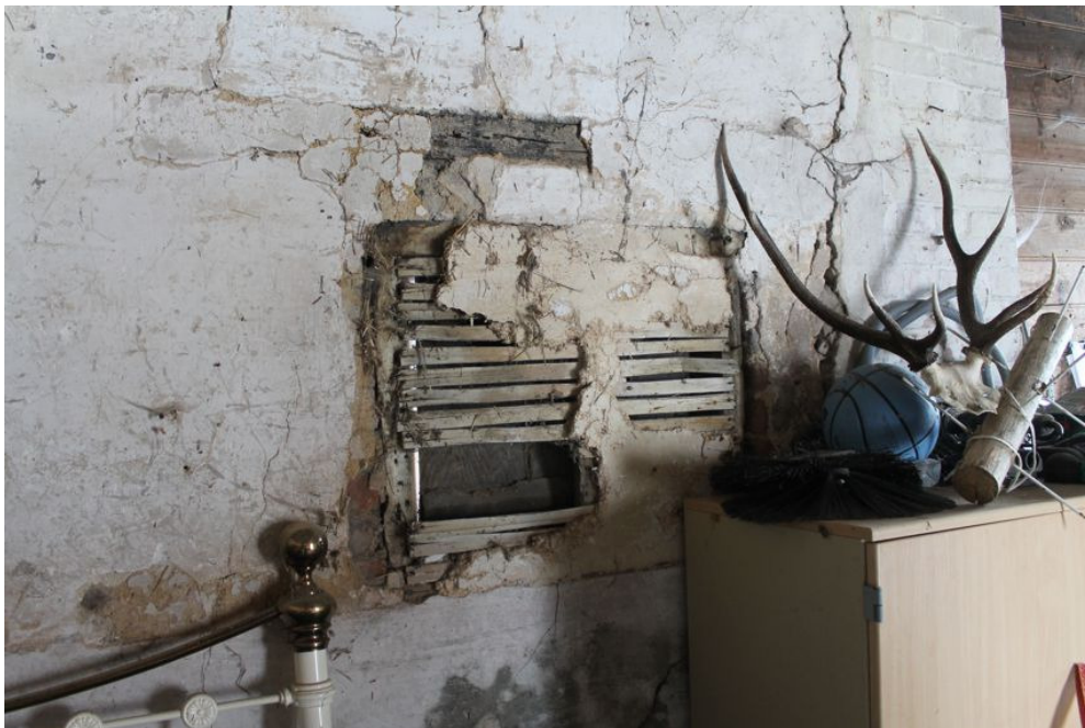
Photograph 9 Partially plastered over hatch from interior of building - looking east.
