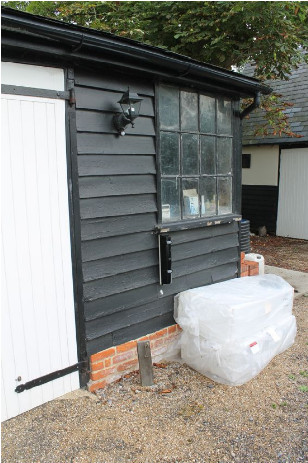
Photograph 6 Detail of twelve-light window on southeast elevation of outshot - looking north.
