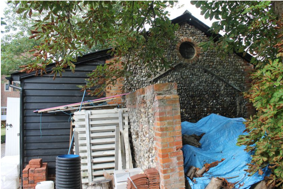
Photograph 4 Northeast elevation of outbuilding and outshot – looking west.
