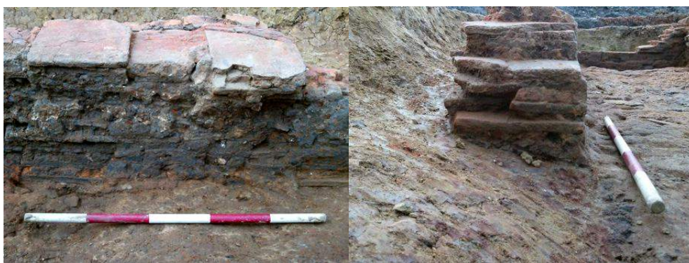
9, 10: burnt inside face of central spine, and end view of western wall.
