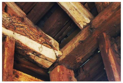
**Photograph 10** Detail of carpenter's mark 'IIII' in east corner of barn. Photograph taken facing east. Contrast increased for better visibility.
