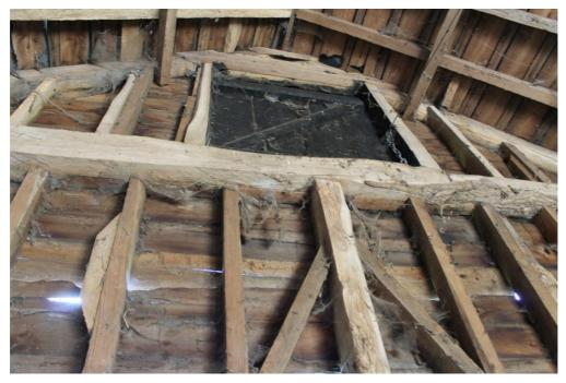
**Photograph 7** Underside of wall plate on north-east elevation of barn, showing machine-cut timber used in repair. Photograph taken facing north-east.
