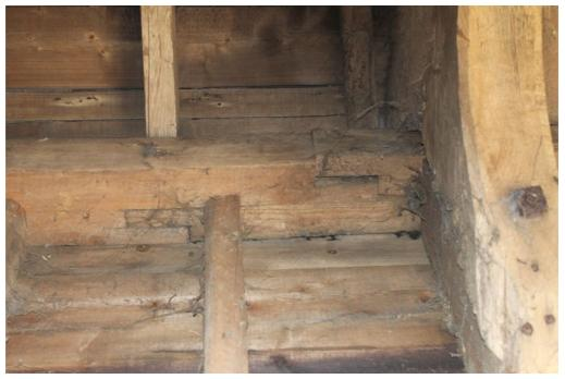
**Photograph 8** Detail of wall-plate on southern end of bay 3, showing scarf joint. Photograph taken facing south-east.
