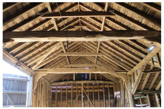
**Photograph 6** Roof of the barn, showing tie-beams and collars. Photograph taken facing south-west.
