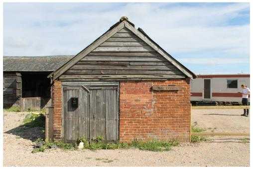
**Photograph 15** South-east elevation of brick outbuilding, showing double-door and blocked in opening. Photograph taken facing north-west.
