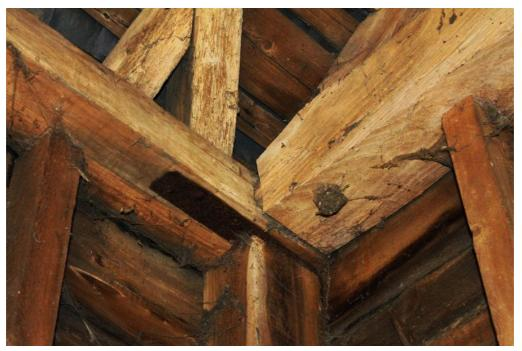
**Photograph 9** Detail of carpenter's mark 'l' in north corner of barn. Photograph taken facing north. Contrast increased for better visibility.
