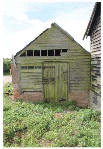
**Photograph 14** North-west elevation of brick outbuilding, showing timber-frame. Photograph taken facing south-east.
