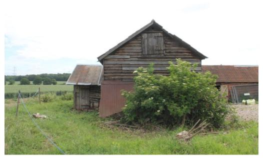
**Photograph 3** South-west elevation of barn, showing pitching door in gable. Collapsed lean-to in foreground. Photograph taken facing north-east.
