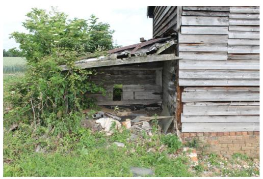
Photograph 19 Partially collapsed lean-to. Photograph taken facing north-west.
