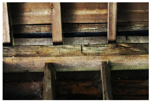
**Photograph 12** Detail of Baltic shipping marks on wall-plate on north-west side of bay 3. Photograph taken facing north-west. Contrast increased for better visibility.
