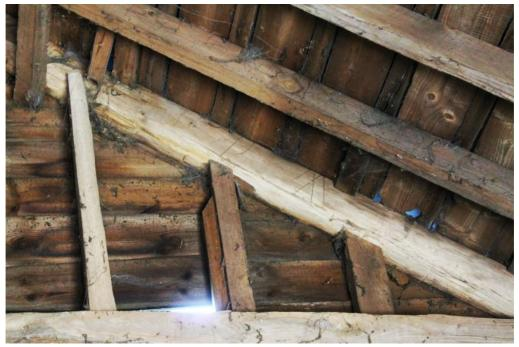
**Photograph 11** Detail of Baltic shipping marks on north-eastern gable end. Photograph taken facing north-east. Contrast increased for better visibility.
