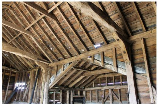
**Photograph 5** North-west side of bay 2, showing wall-plate and two machine-cut principal posts. Photograph taken facing west.
