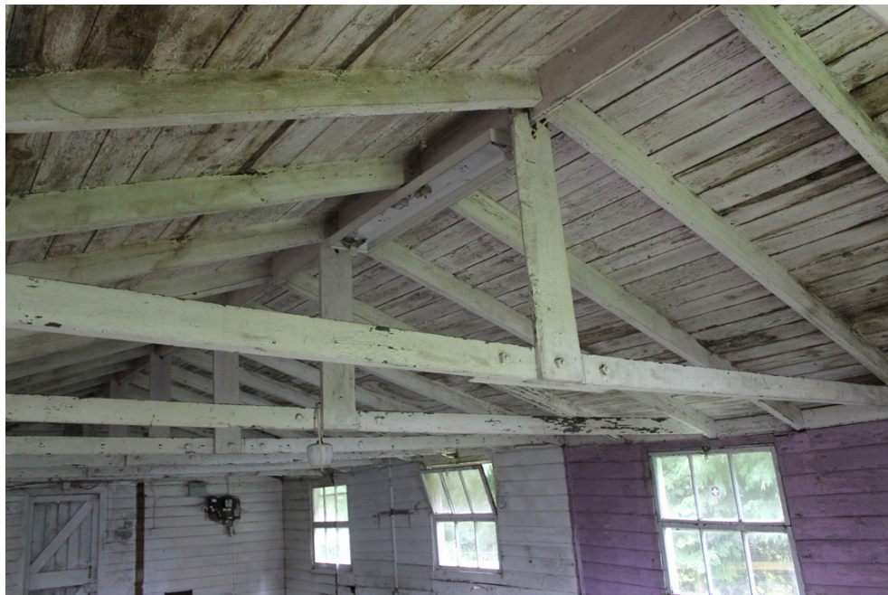
Photograph 6 King-post roof trusses. Photograph taken facing south-east.
