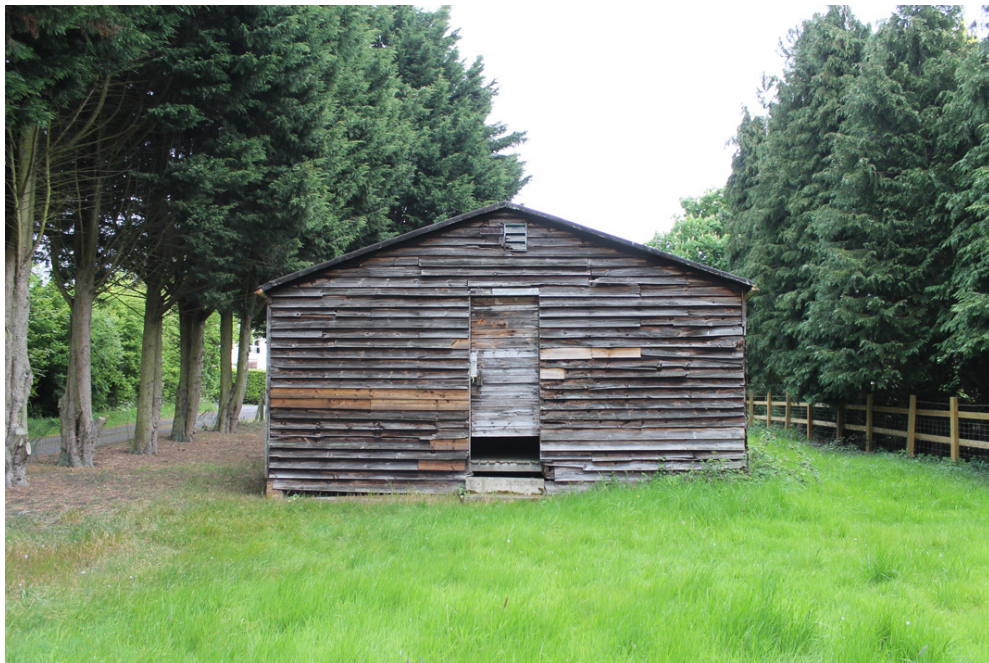
Photograph 4 West elevation of Mission Hall. Photograph taken facing east.
