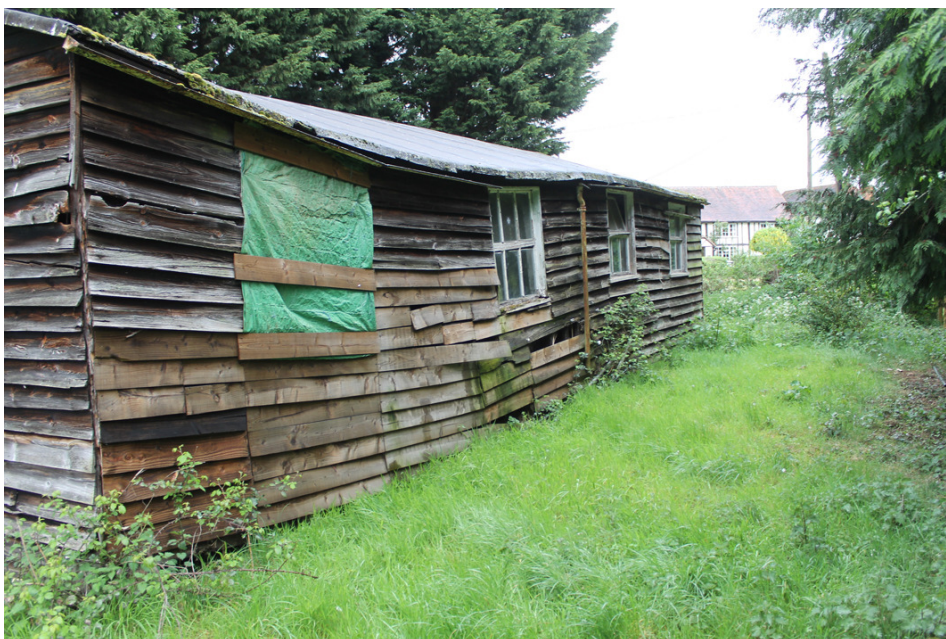
Photograph 2 South elevation of Mission Hall. Photograph taken facing north-east.
