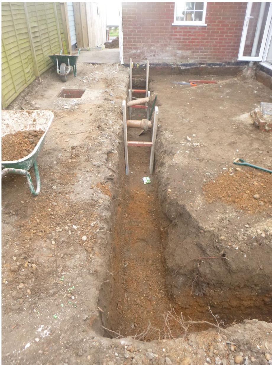
Photograph 1 Foundation trenches, looking SW
