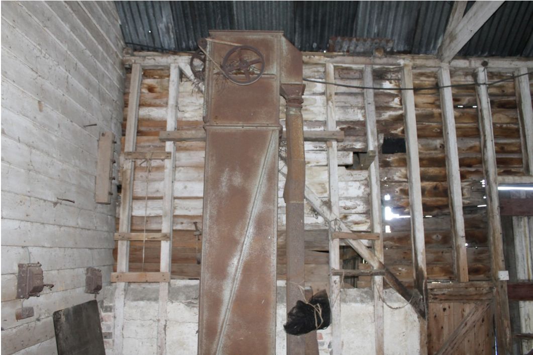
Photograph 27 North-west framing of bays 8 and 7 showing the frame built up against the exterior of bays 9 and 10. The primary bracing crosses both bays. The machinery is a grain hoist and probably dates to the mid 20th century – view west.
