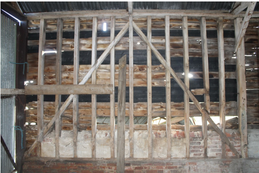
Photograph 12 South-east framing to bays 1 and 2 - view south-east.
