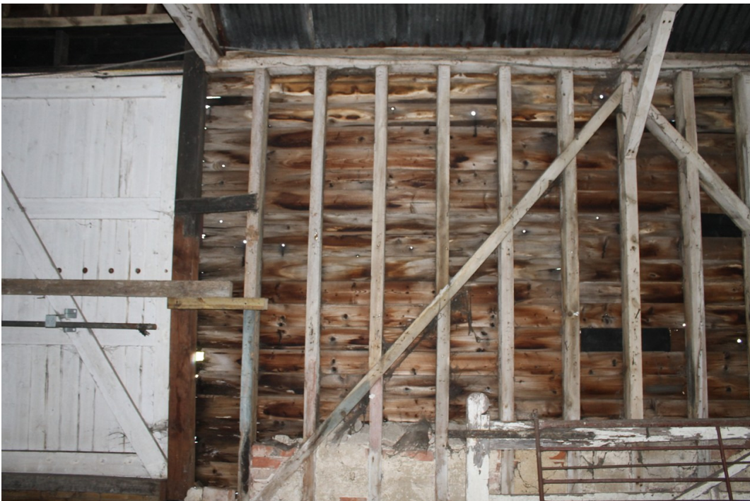
Photograph 20 North-west framing of bay 5 – view north-west.
