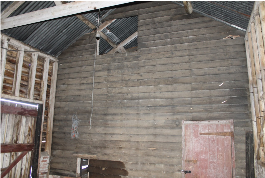
Photograph 24 Weatherboard to exterior face of bay 6, viewed from bay 7, with the frames of the 19th-century extension built up against the main barn and raised on taller brick plinths – view north.
