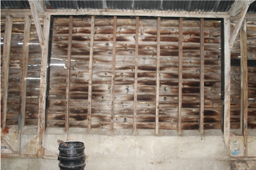
Photograph 21 South-east framing of bay 6 replacing original cart door opening – view south-east.
