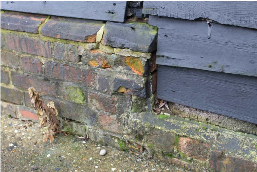
Photograph 2 North-west elevation, showing plinth of main barn to the left with 19th-century extension to the right built on a much shallower plinth - view north-east.
