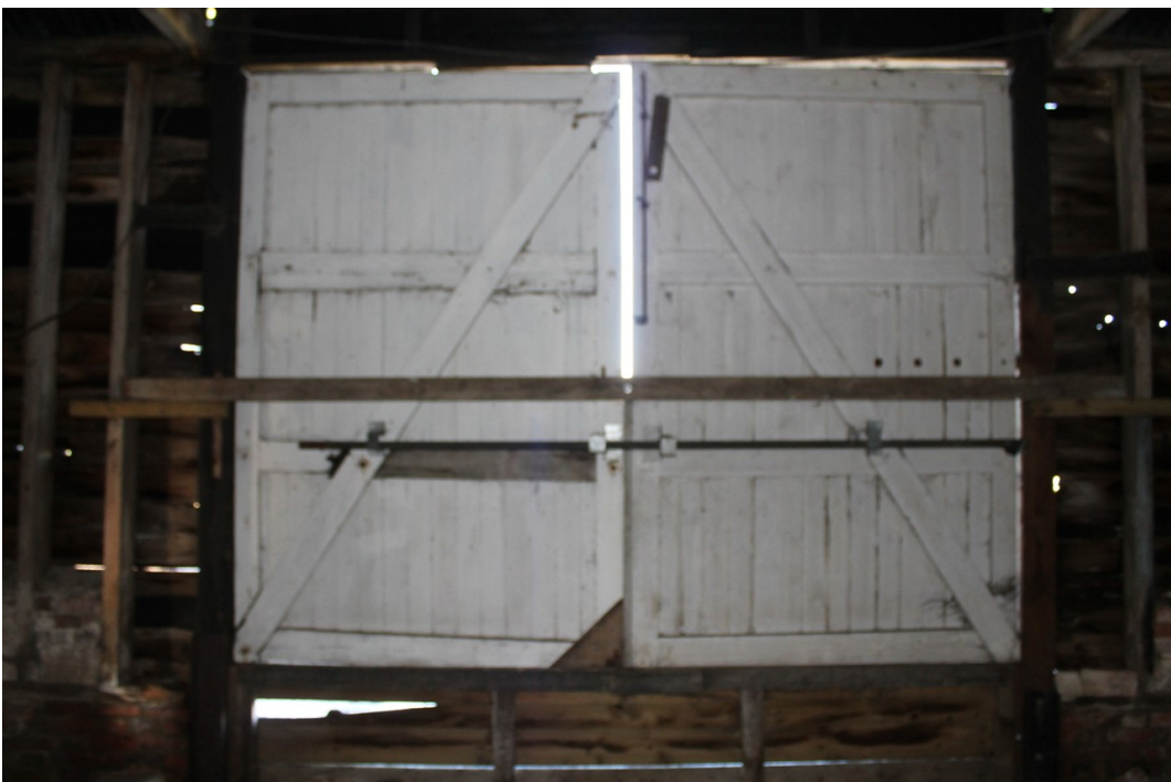
Photograph 22 Replacement cart doors to original midstrey in bay 6 – view north-west.
