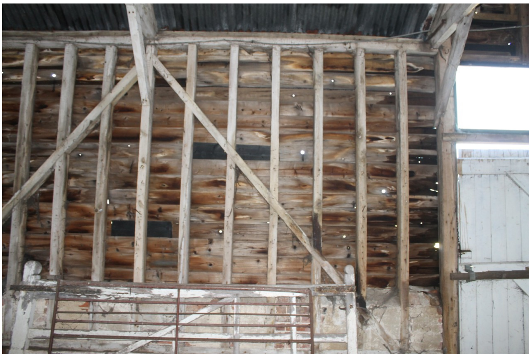
Photograph 18 North-west framing to bay 4 – view north-west.
