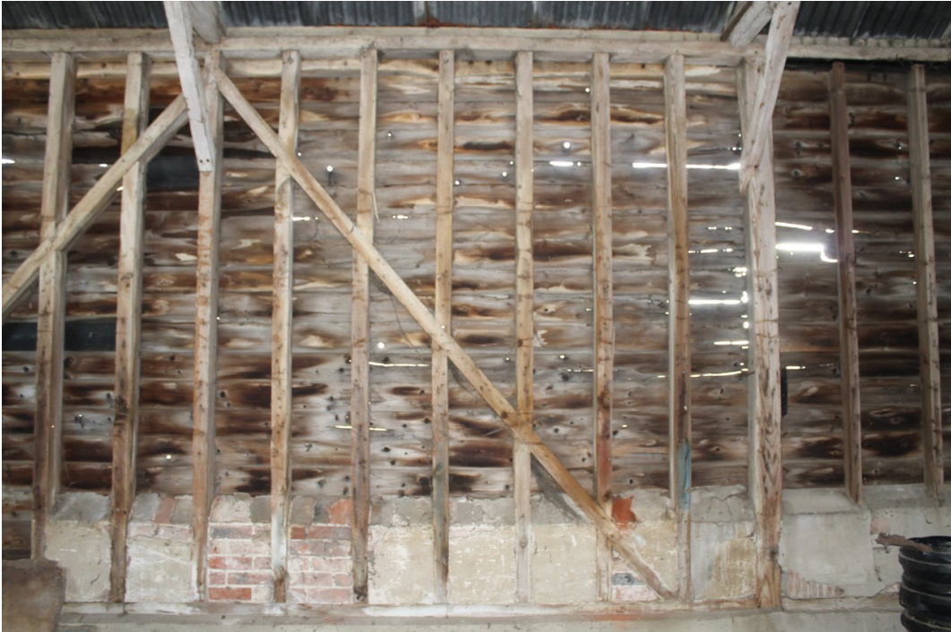
Photograph 19 South-east framing to bay 5 – view south-east.
