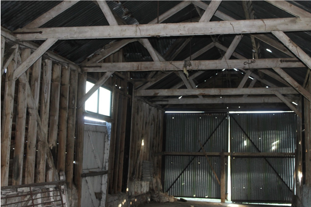
Photograph 9 Interior of the 18th-century barn, with the partially blocked midstrey of bay 3 to the left and the 20th-century doors replacing the north gable frame – view north.
