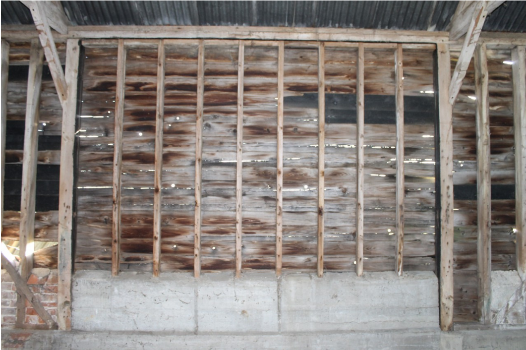
Photograph 15 South-east framing to bay 3 replacing original cart door opening - view south-east.
