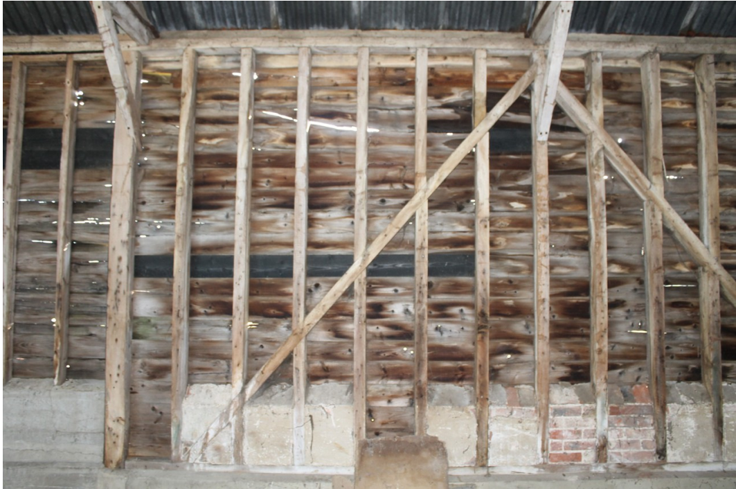
Photograph 17 South-east framing to bay 4 – view south-east.
