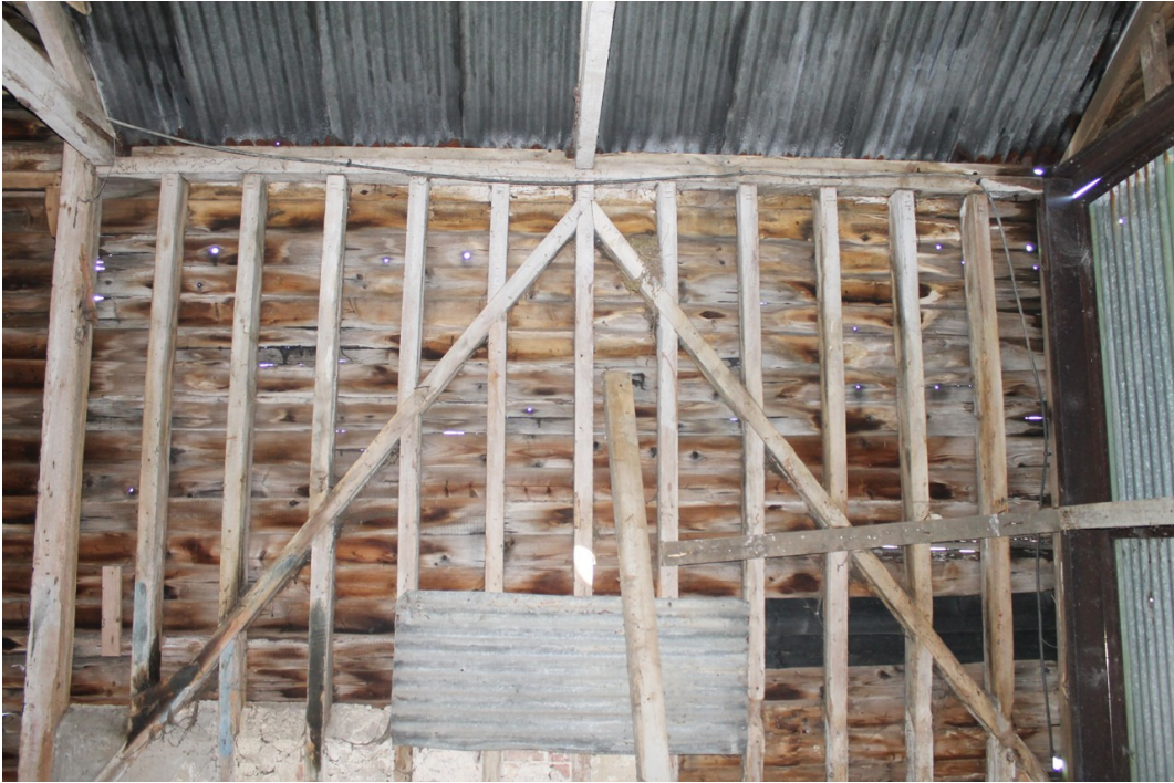
Photograph 13 North-west framing to bays 2 and 1- view north-west.
