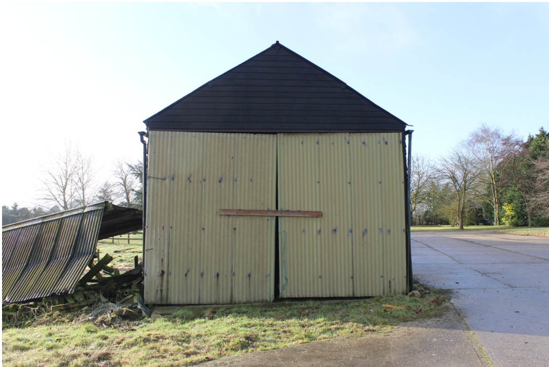
Photograph 7 North-east elevation of the 18th-century barn with modern full height doors formed from galvanised sheets over steel frames; the ruins of OB2 are on the left - view south-west.
