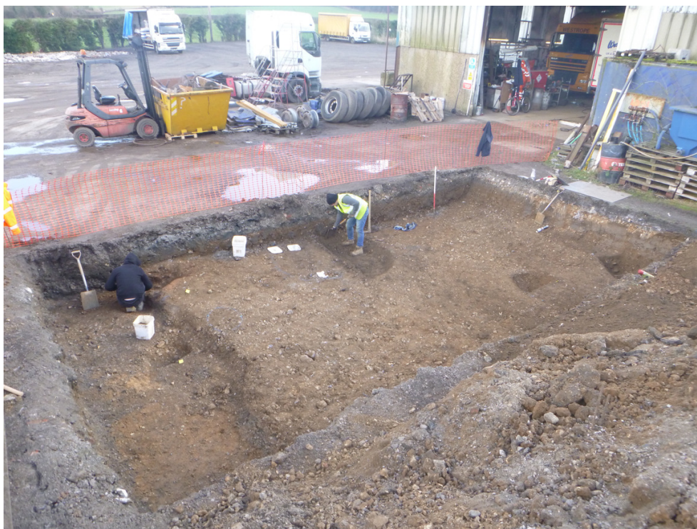
Photograph 1 General site shot, looking south
