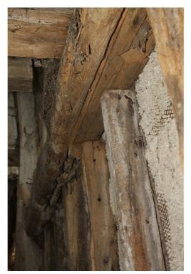
**Photograph 7** Underside of girding beam on west side of bay one. Window mullions and shutter grooves visible. Photo taken facing south-west.
