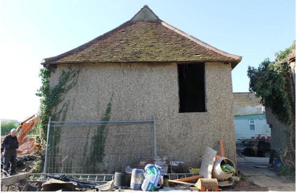
**Photograph 2** Northern exterior elevation of barn, showing inserted pitching door and gablet roof. Photo taken facing south.
