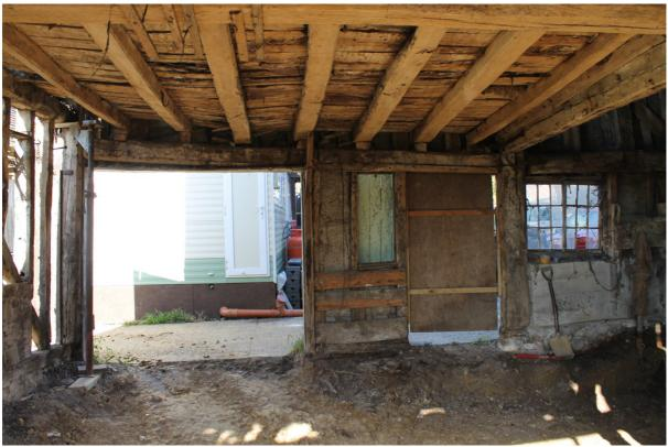
**Photograph 18** West side of bay three, lower register. Modern doorways and windows into barn visible. Photo taken facing west.
