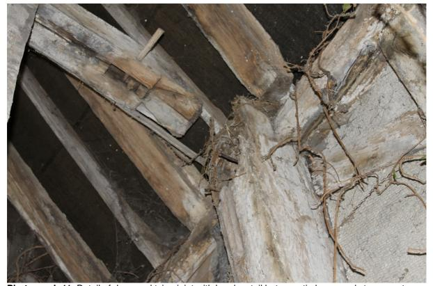
**Photograph 11** Detail of damaged tying joint with lap dovetail between tie beam and storey post on eastern elevation. Photo taken facing north-east.
