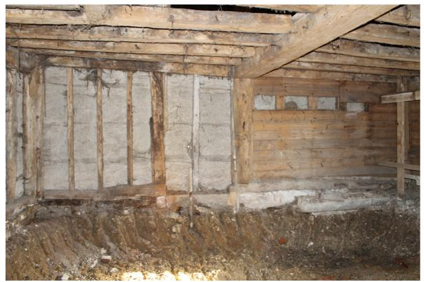
**Photograph 4** North side of bay one, lower register. Blocked inserted doorway visible. Photo taken facing north.
