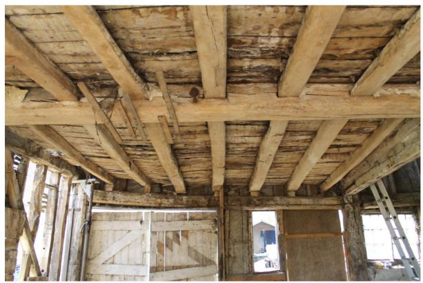
**Photograph 21** Underneath of first floor in bay three, showing joists supported by offcut pieces of timber on west side. Photo taken facing west.
