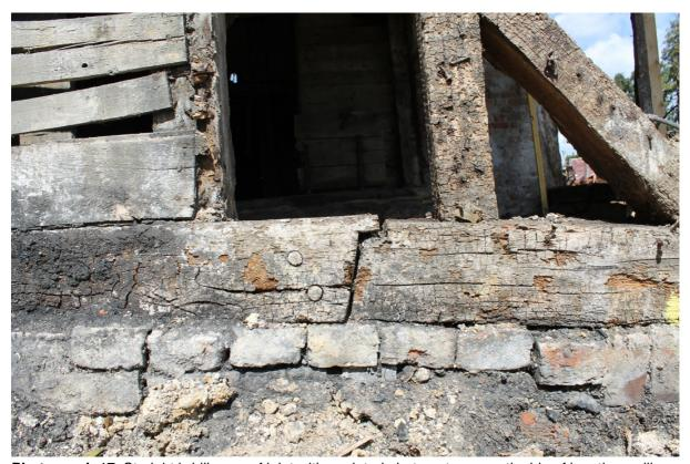
**Photograph 17** Straight bridling scarf joint with squinted abutments on south side of bay three sill beam. Photo taken facing north.
