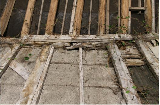
**Photograph 13** Detail of snapped face-halved scarf joint on east side of bay two wall plate. Photo taken facing east.
