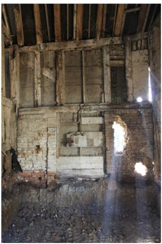
**Photograph 12** East side of bay two. Brick infill and modern repair visible. Photo taken facing east.
