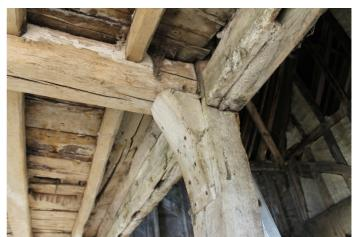
**Photograph 20** North side of bay three, showing binding beam of first floor jointed to storey post and supported with a knee brace. Photo taken facing north-west.
