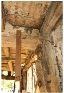
Photograph 19 South side of bay three, showing binding beam of first floor jointed to storey post. Photo taken facing east.
