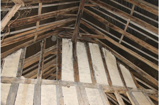
**Photograph 24** Detail of crown-post roof truss and dividing wall with wattle-and-daub infill between bays one and two. Photo taken facing north.
