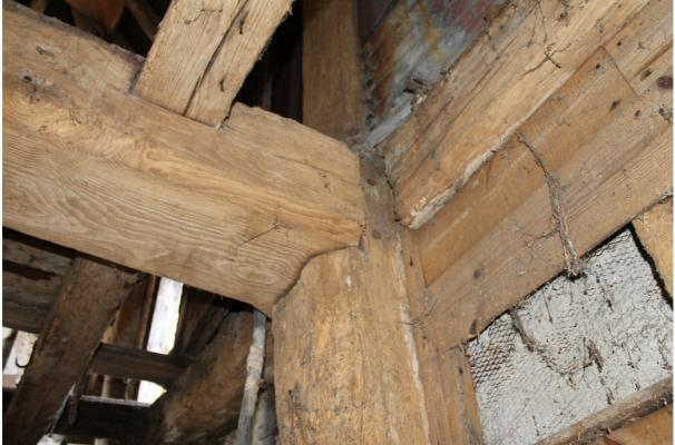
**Photograph 9** North side of bay one, showing binding beam for first floor jointed to storey post. Photo taken facing north-west.
