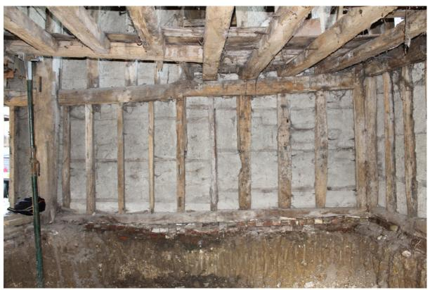
**Photograph 6** West side of bay one, lower register. Modern and reused timbers visible as studs. Natural curve on girding beam visible. Photo taken facing west.
