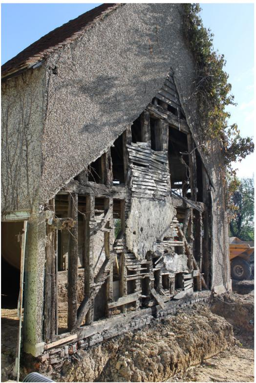
**Photograph 5** Southern exterior elevation of barn. Scar in location of recently demolished outbuilding visible, exposing timber-frame. Photo taken facing north-east.
