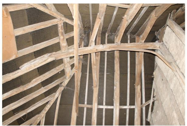
**Photograph 23** Detail of roof timbers at northern end of barn by rebuilt gablet. Scarf joint in collar purlin visible. Photo taken facing east.
