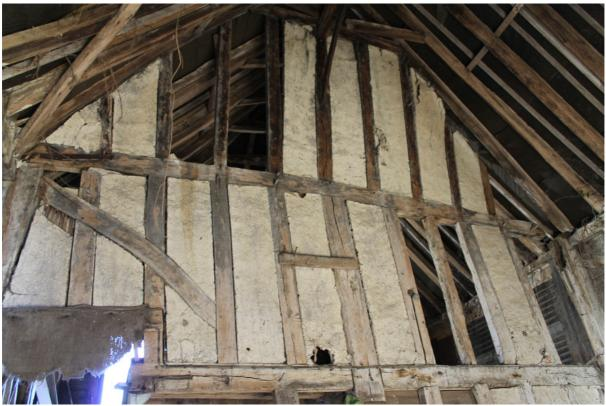
**Photograph 10** North side of bay two, upper register. Showing wattle and daub infill between studs. Photo taken facing north.
