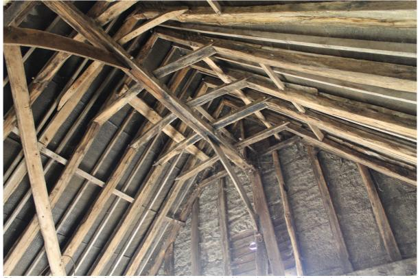
**Photograph 22** Detail of roof timbers at southern end of barn by gable. Photo taken facing southeast.
