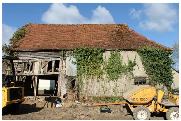
**Photograph 3** Eastern exterior elevation of barn, showing brick repairs to bay two and removed timbers in bay three. Photo taken facing west.
