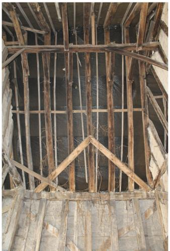
Photograph 15 West side of bay two, upper register and roof detail, showing modern reinforcing timbers. Photo taken facing south.
