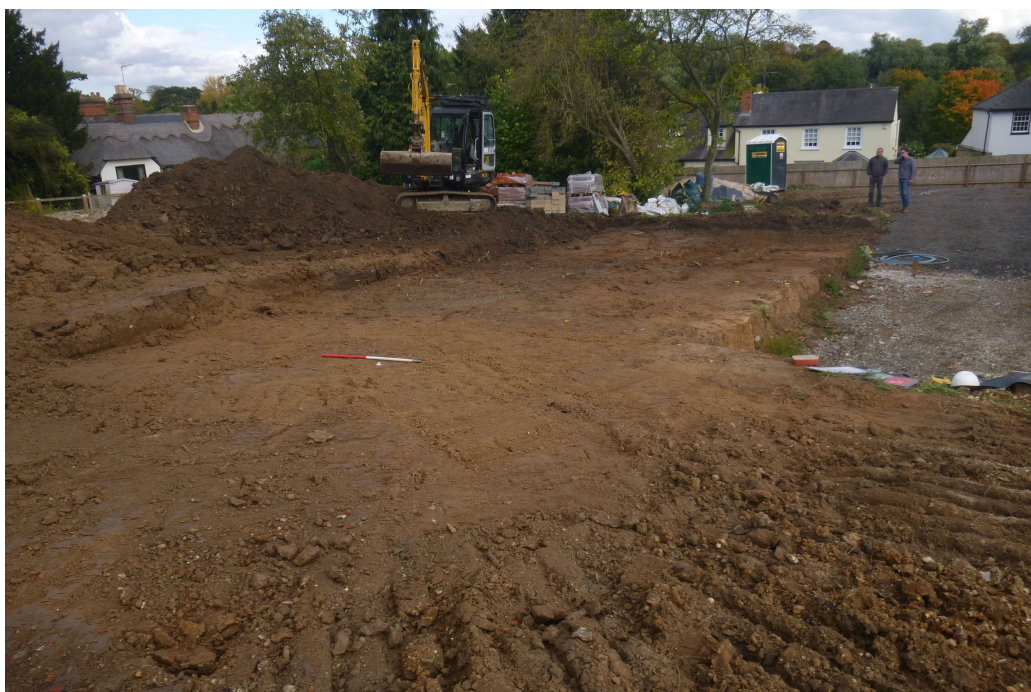
Photograph 2 Cartlodge strip, looking ENE
