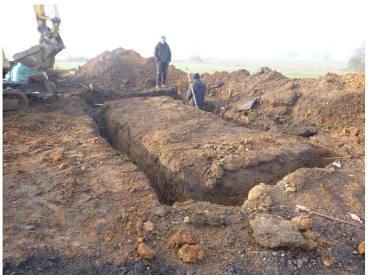
Photograph 2 Garage: foundation trenches fully excavated, looking NW
